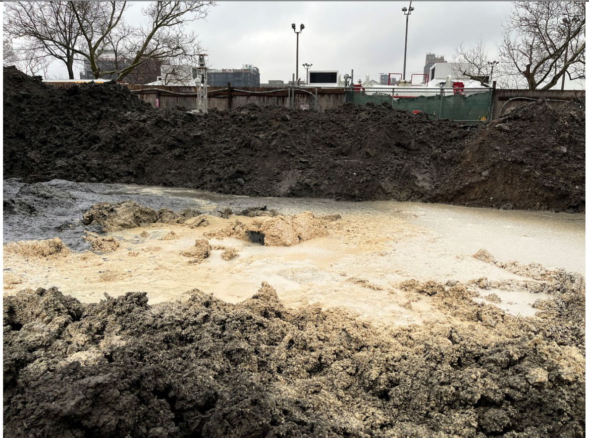
Photo 3- Representative photo of ATMOS foam sprayed over swell material.
