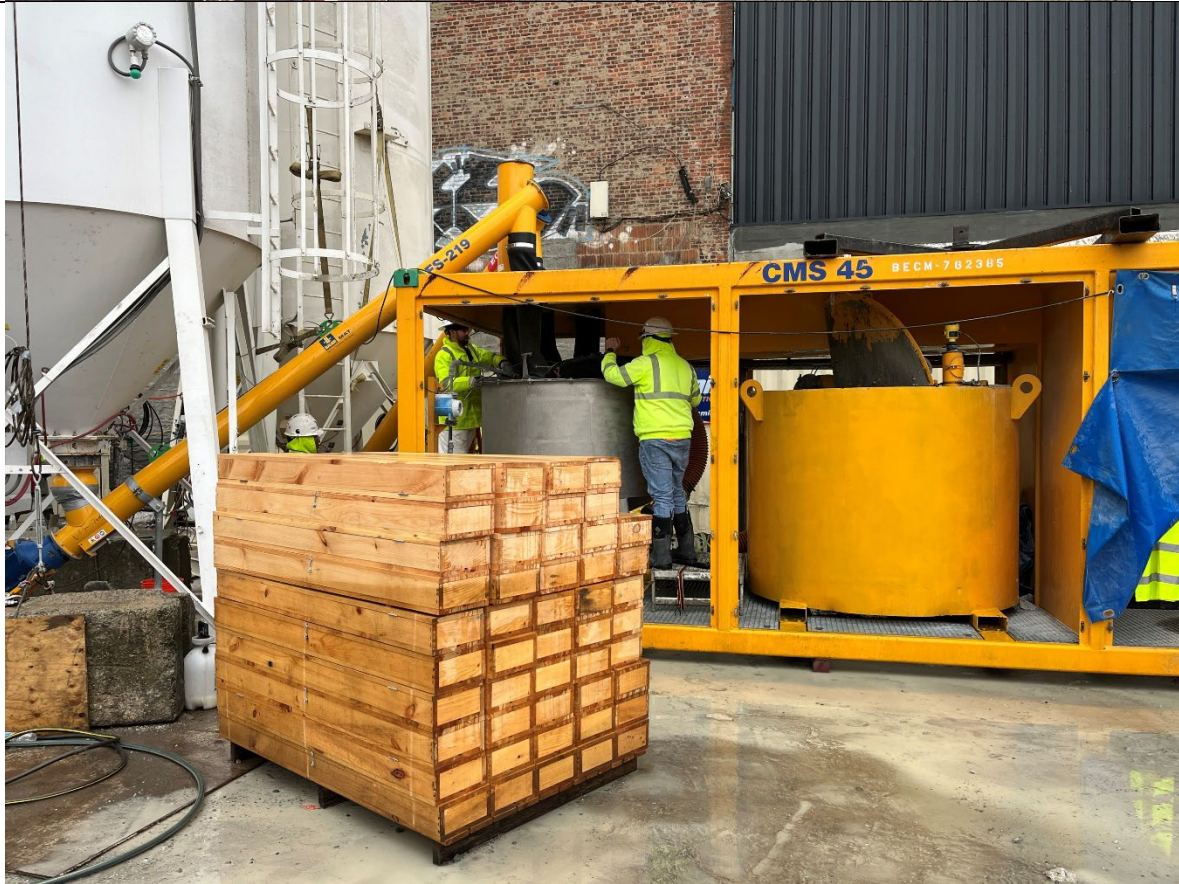
Photo 2- Representative photo of Cascade working to unclog slag chute.
