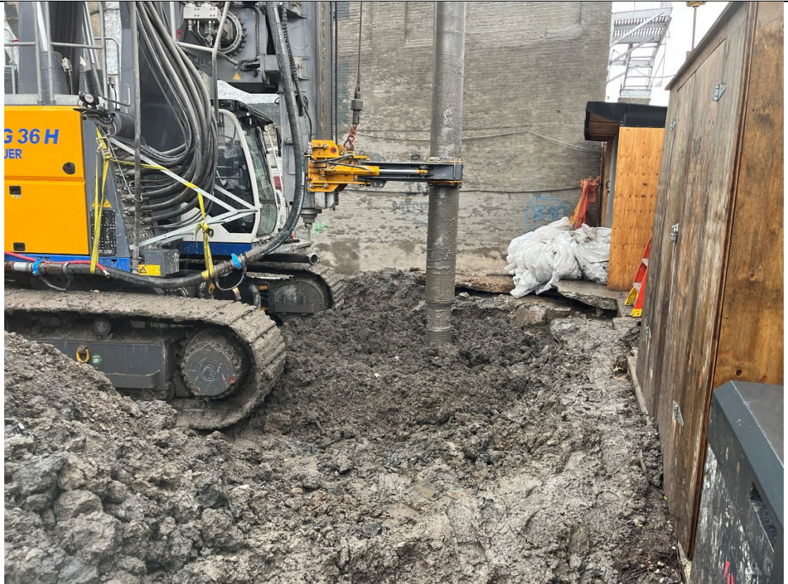
Photo 5- Representative photo of drilling an ISS column.
