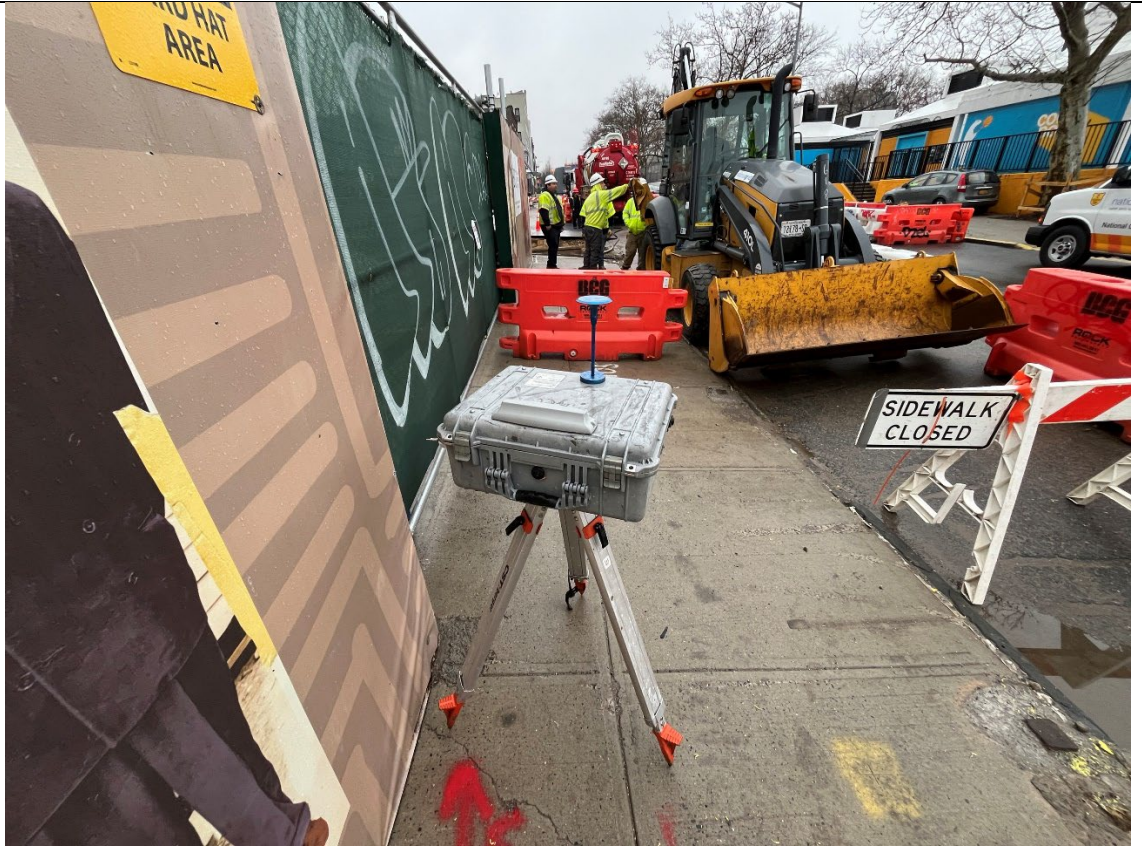
Photo 1- Representative photo of Downwind 1 CAMP unit positioned for sidewalk work
