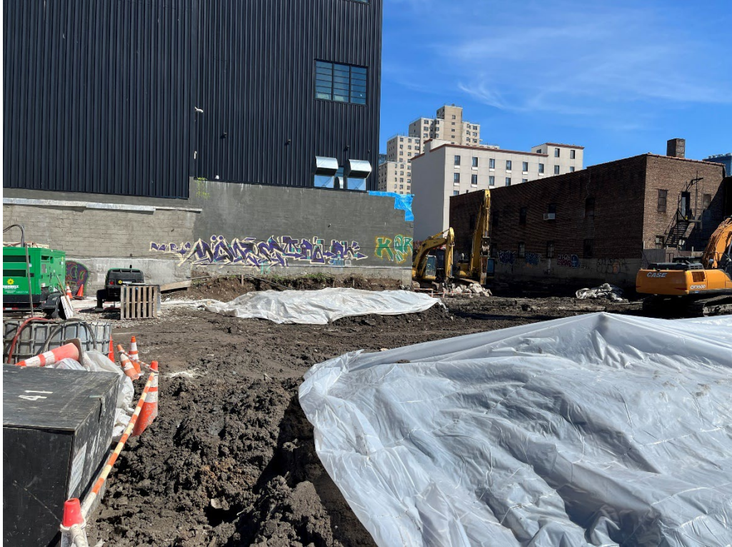
Photo 6- Additional representative photo of stockpiled swell material covered at the end of day.
