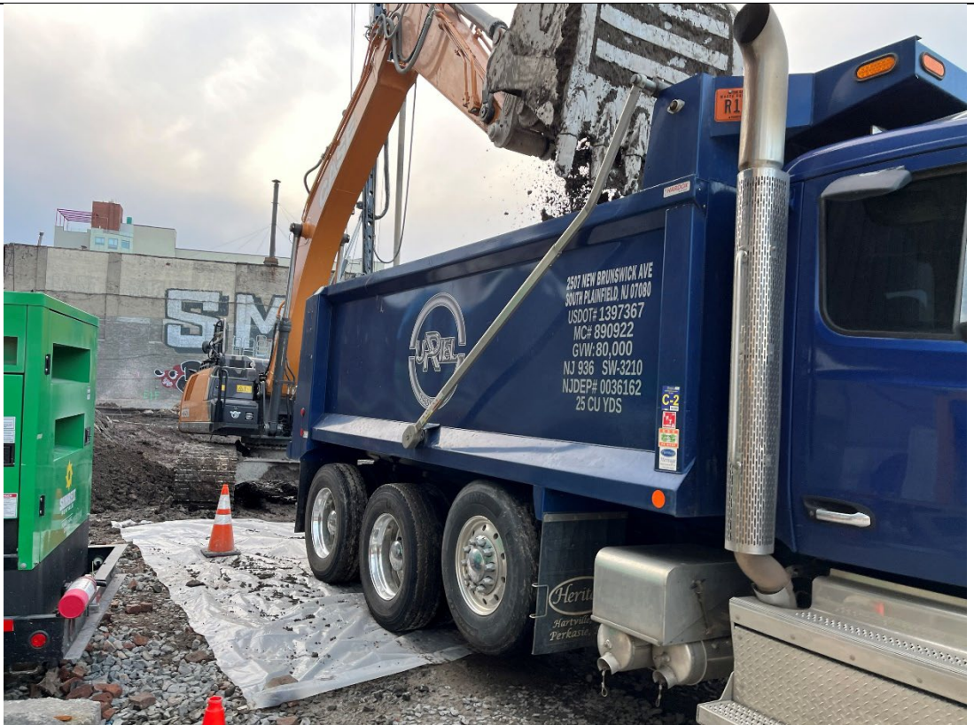
Photo 4- Representative photo of swell material being loaded for disposal offsite.
