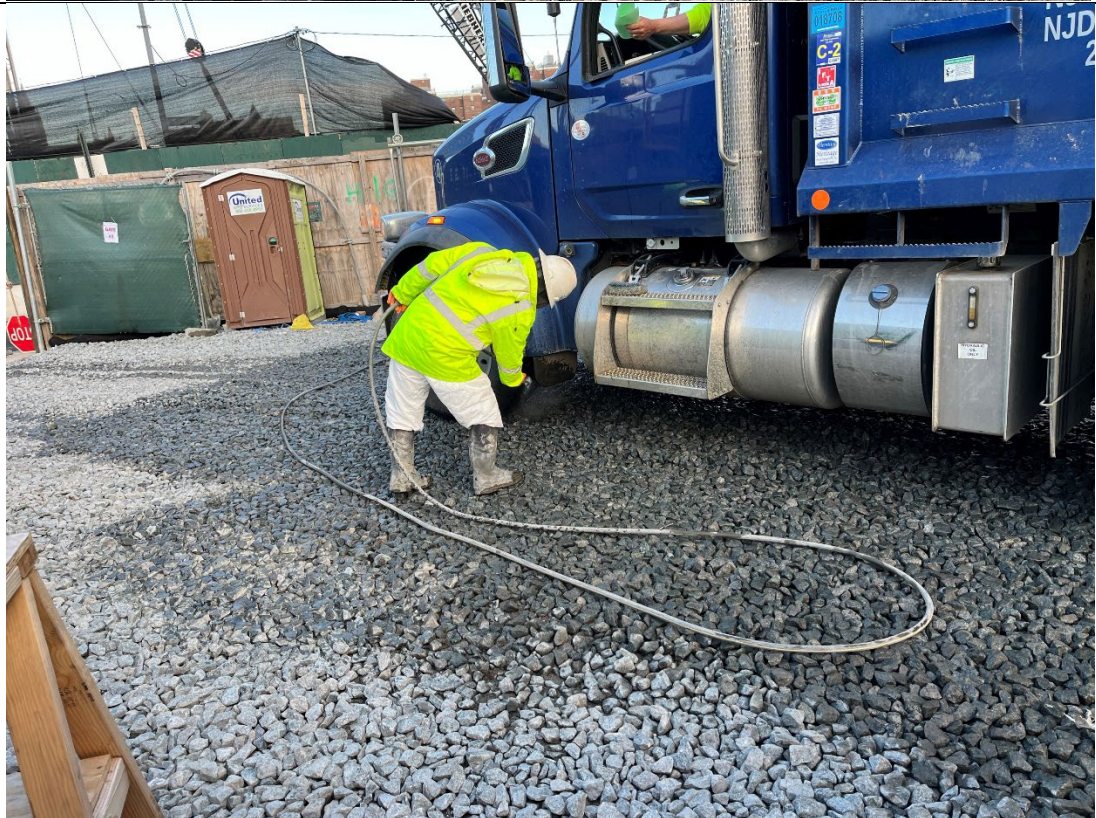
Photo 2- Representative photo of truck tires being washed over track pad.
