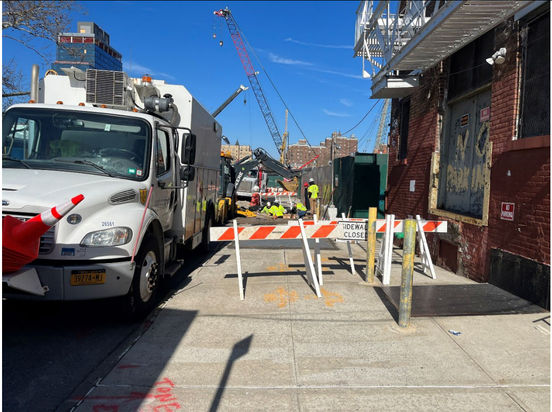
Photo 3- Representative photo of National Grid work in the sidewalk.
