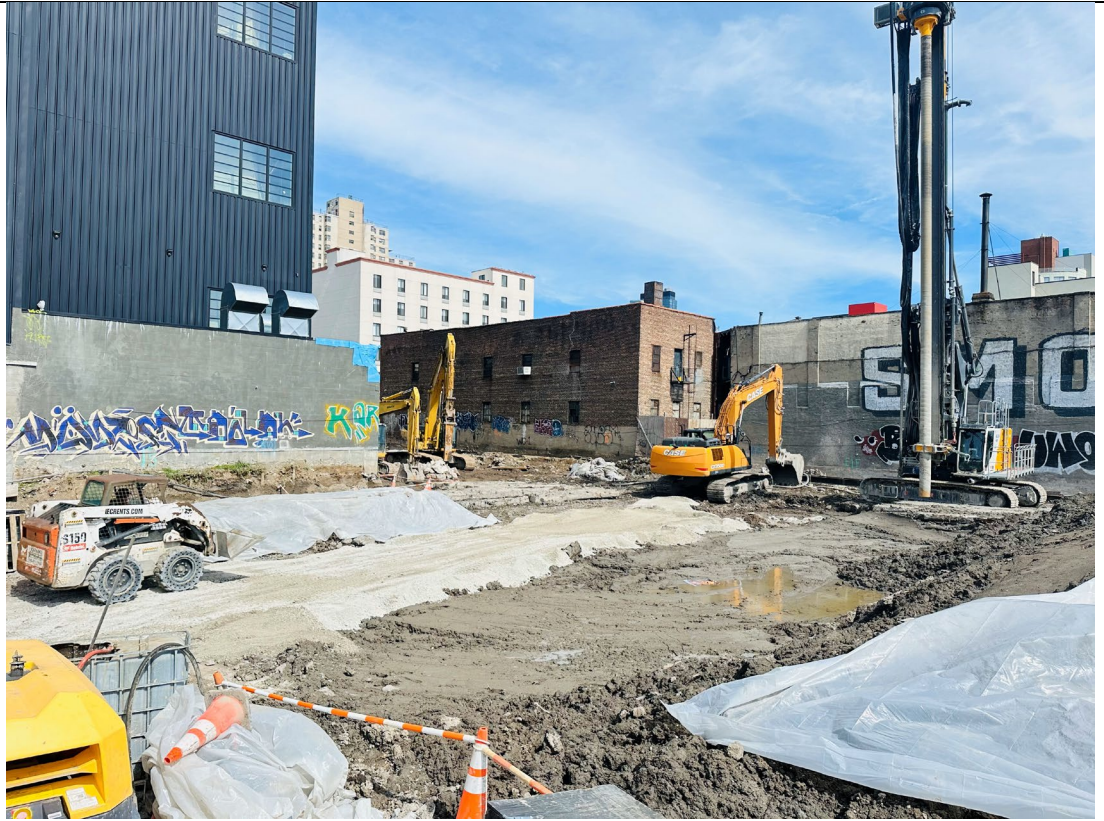
Photo 5- Representative photo of approved stone being placed to create equipment pathway.
