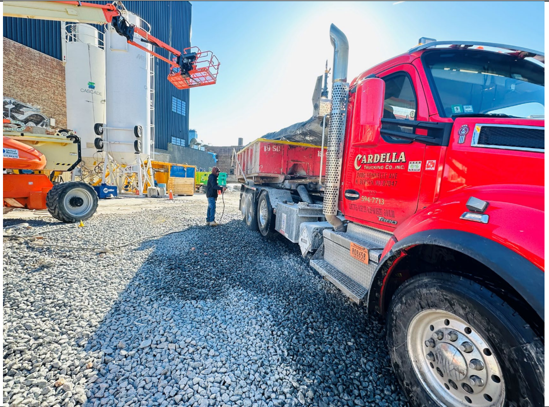
Photo 3- Representative photo of truck tires being washed off over track pad.
