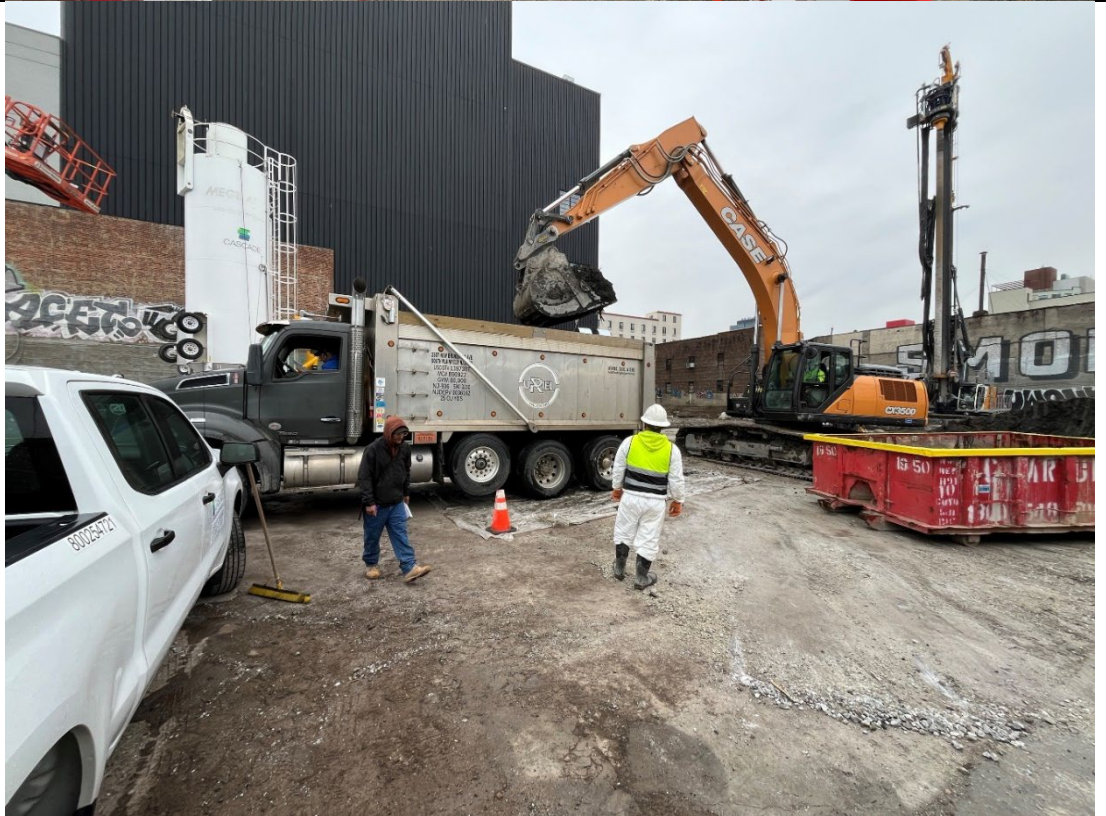
Photo 2- Representative photo of swell material loadout.
