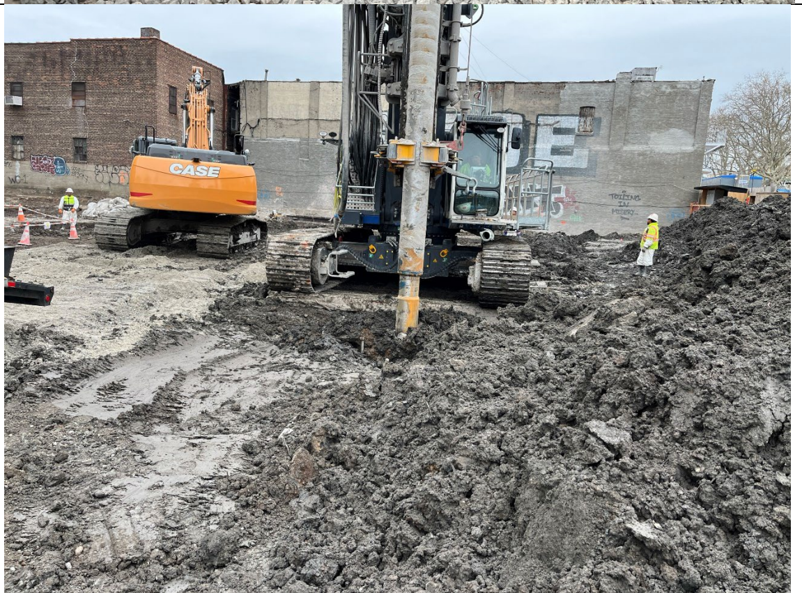
Photo 4- Representative photo of drilling ISS column.
