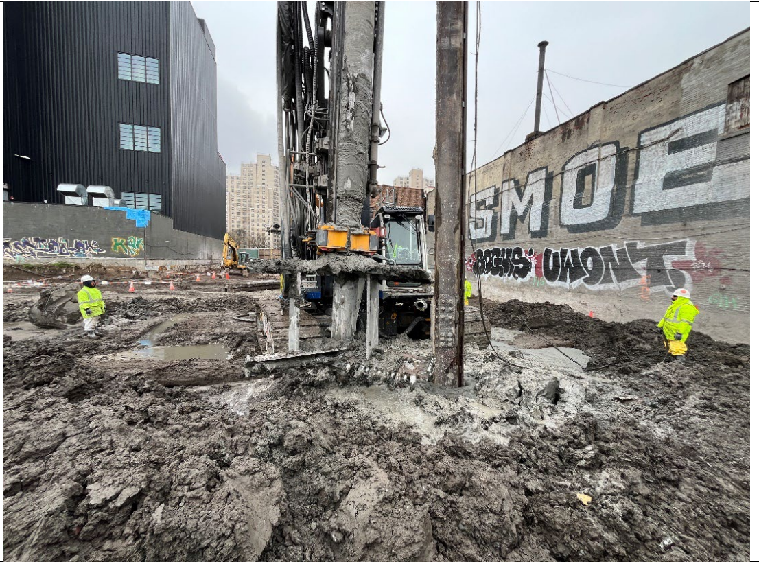
Photo 1- Representative photo of sampling rod at column 9.
