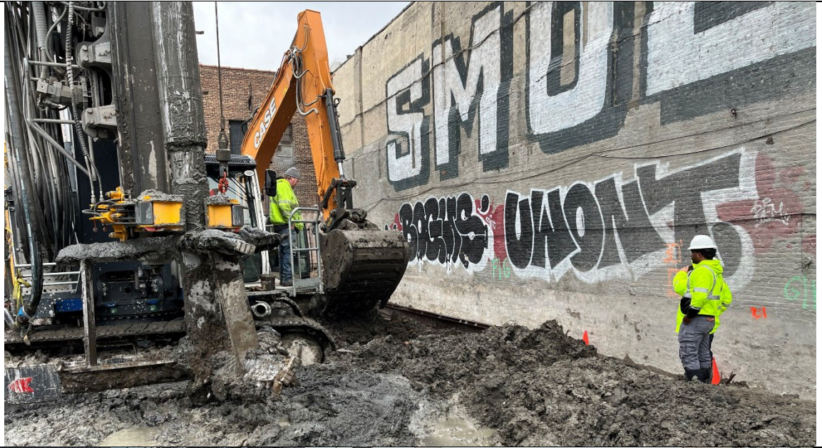
Photo 3- Representative photo of obstruction removal at 4' below grade surface for Column 162.
