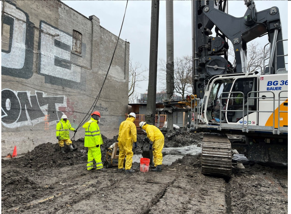
Photo 2- Representative photo of Cascade collecting wet mix sample.
