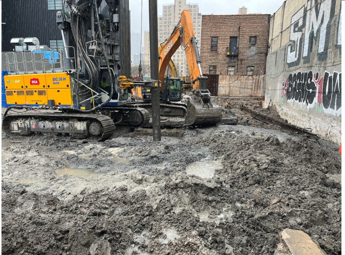
Photo 4- Representative photo of drilling ISS column.
