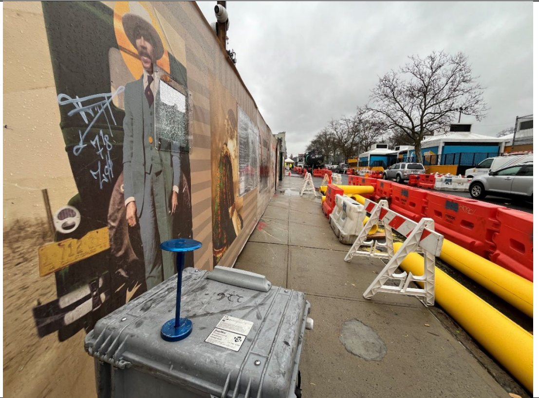
Photo 5- Representative photo of CAMP unit on Douglass Street sidewalk.
