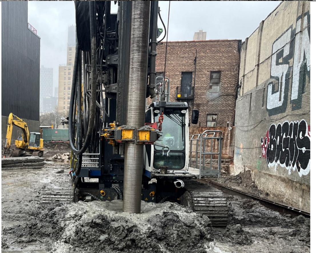
Photo 4- Representative photo of drilling ISS column.
