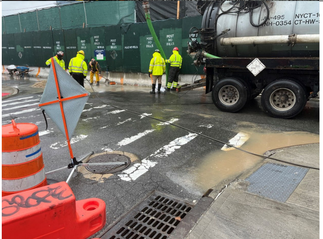
Photo 2- Representative photo of vacuum truck on Nevins Street removing material spilled from adjacent site.
