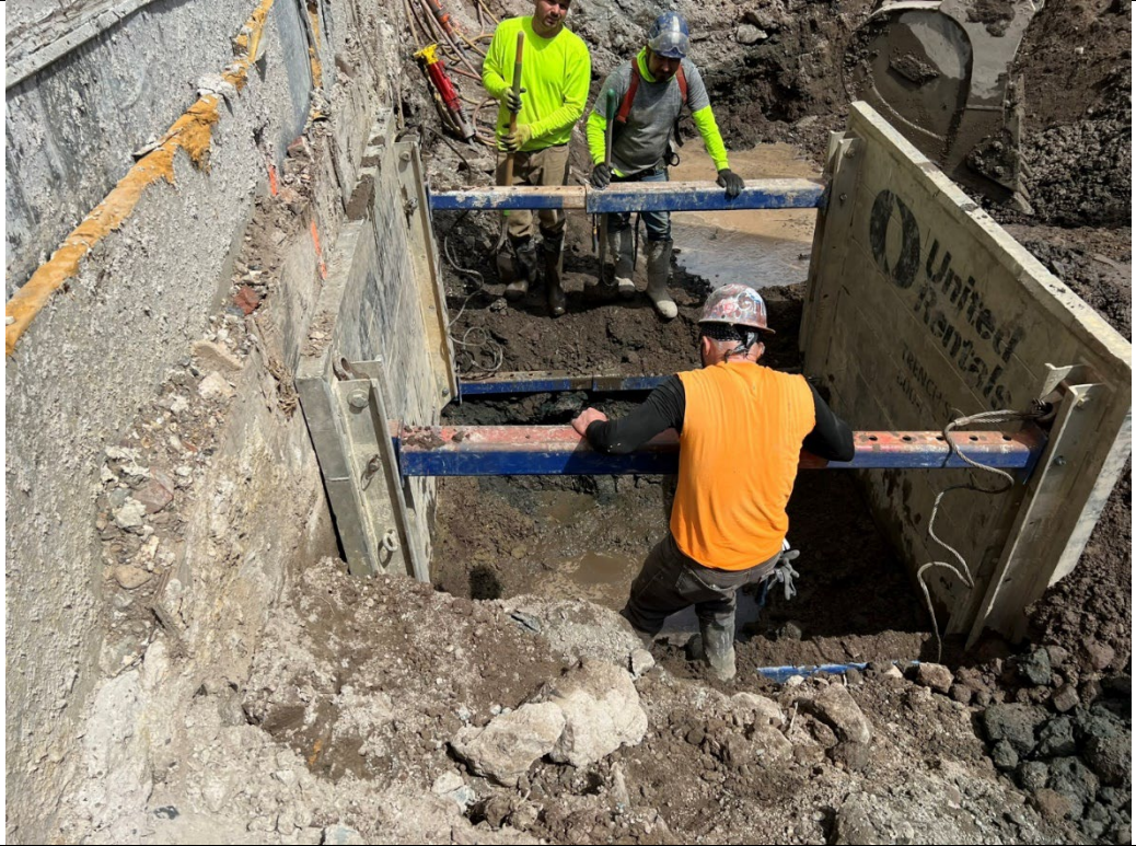
Photo 1- Representative photo of preparing to remove obstruction in the northern alley.
