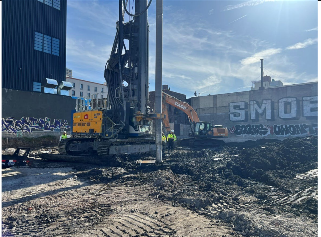
Photo 2- Representative photo of drilling ISS column.
