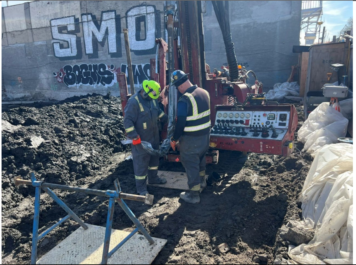
Photo 3- Representative photo of ADT coring a pilot test column.
