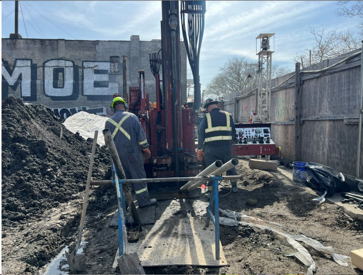
Photo 3- Representative photo of ADT coring a column.
