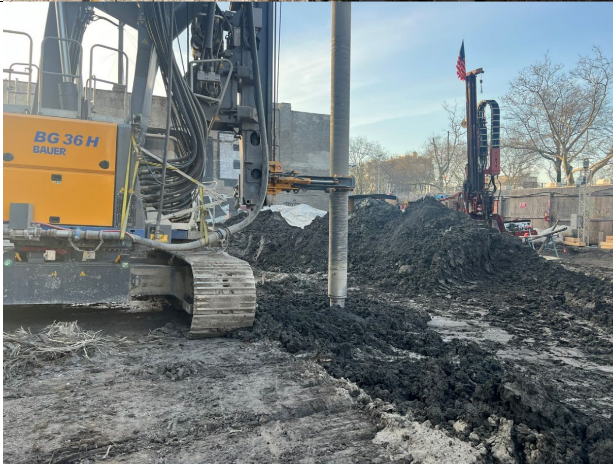
Photo 2- Representative photo of drilling ISS column.
