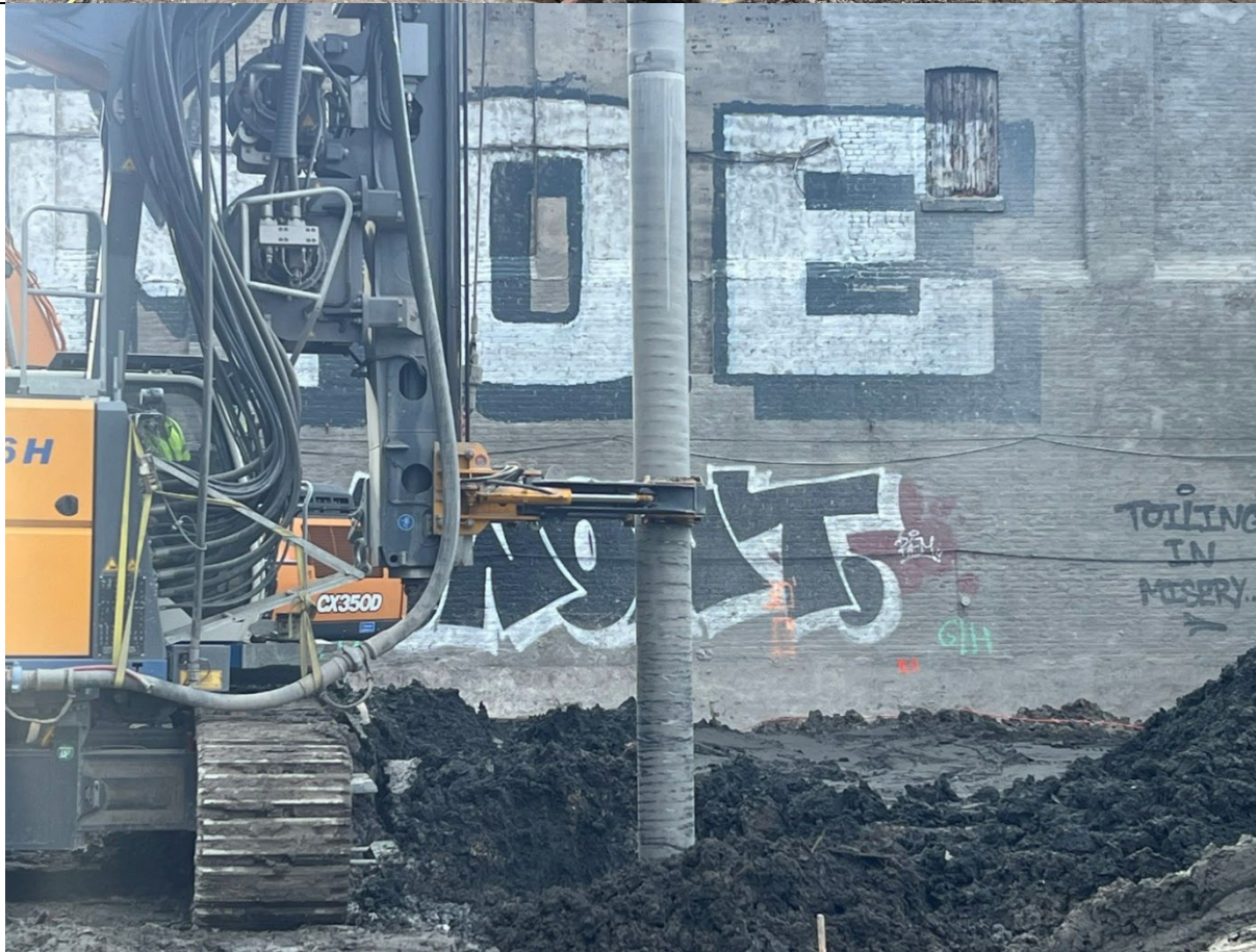
Photo 2- Representative photo of drilling ISS column.
