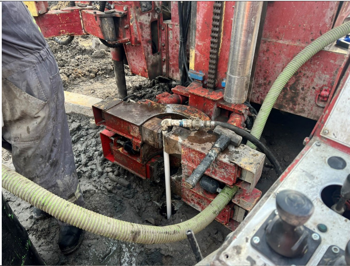
Photo 3- Representative photo of ADT grouting a cored column.
