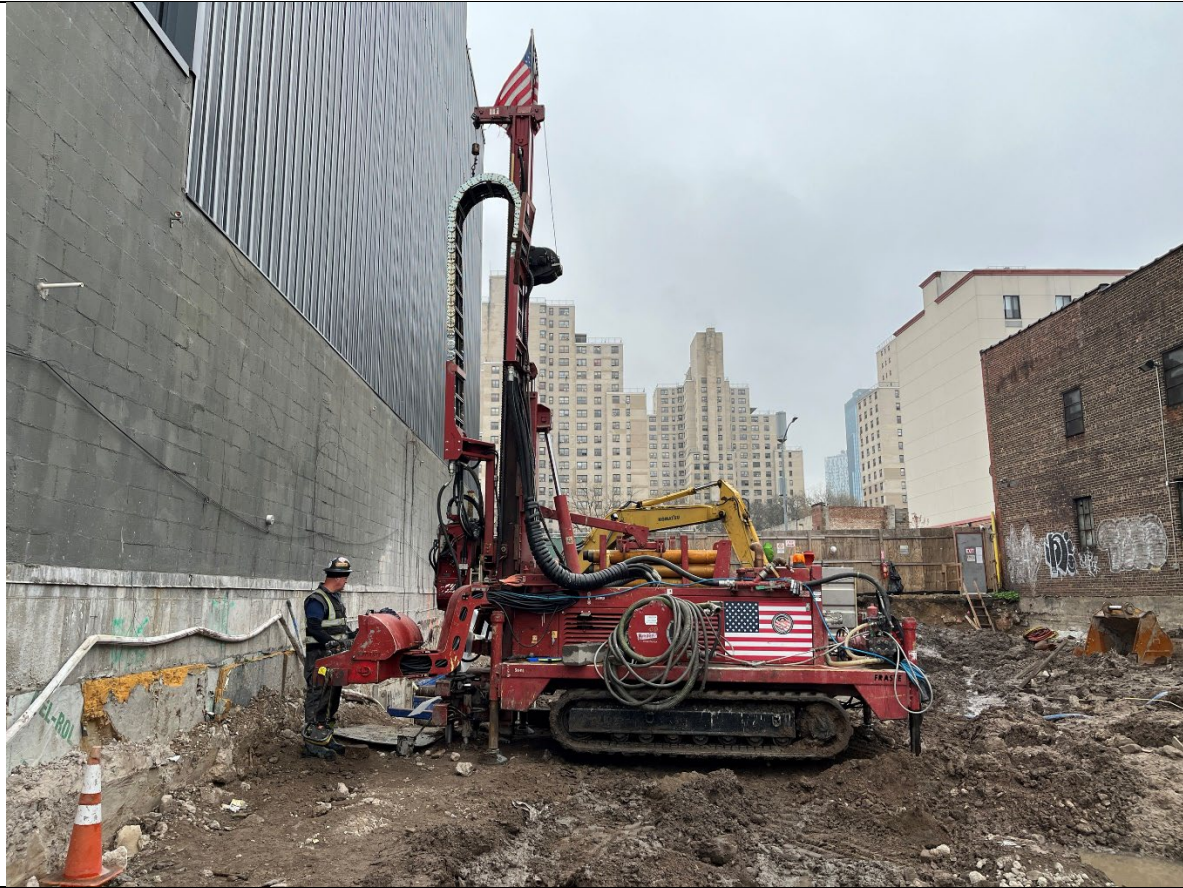
Photo 3- Representative photo of coring a column.
