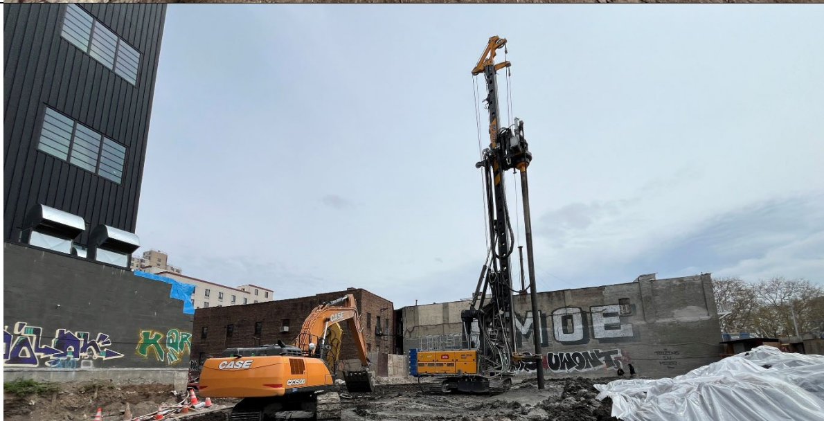
Photo 2- Representative photo of drilling ISS column.
