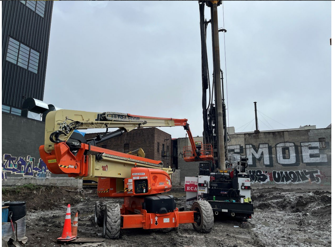
Photo 4- Representative photo of drill rig maintenance by ECA.
