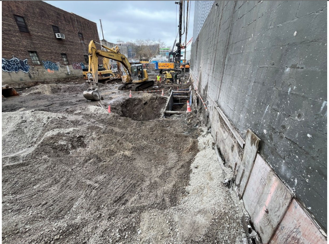
Photo 1- Representative photo of removing the obstruction in the northern alley.
