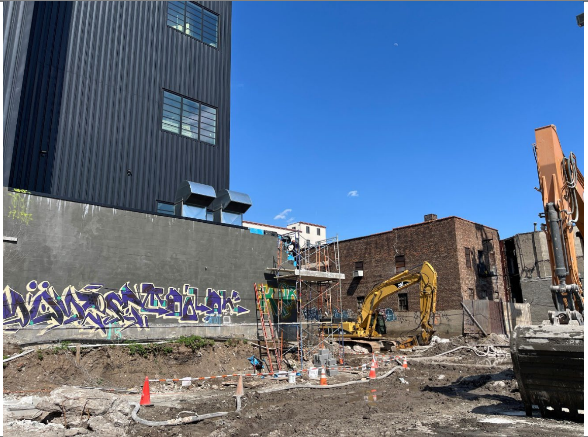
Photo 1- Representative photo of roof repair to adjacent building.
