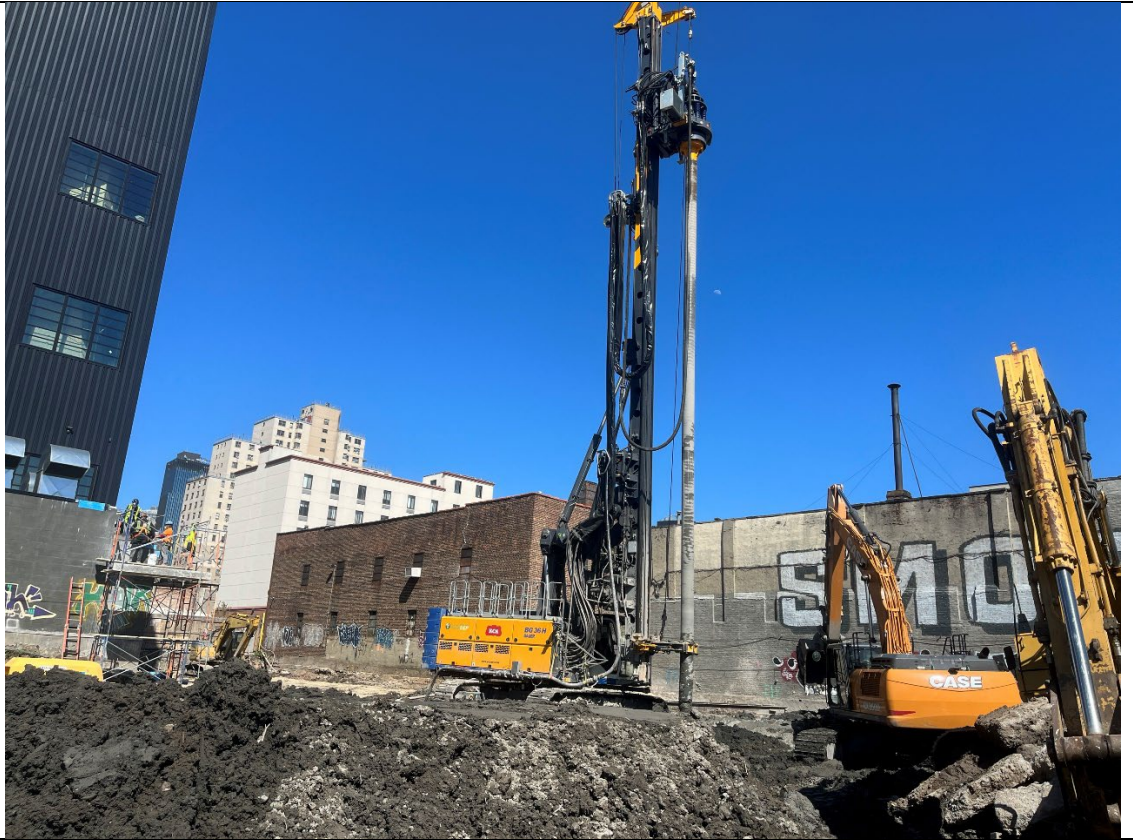
Photo 1- Representative photo of ISS column installation.
