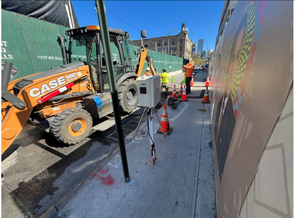
Photo 2- Representative photo of Empire working on Nevins Street.
