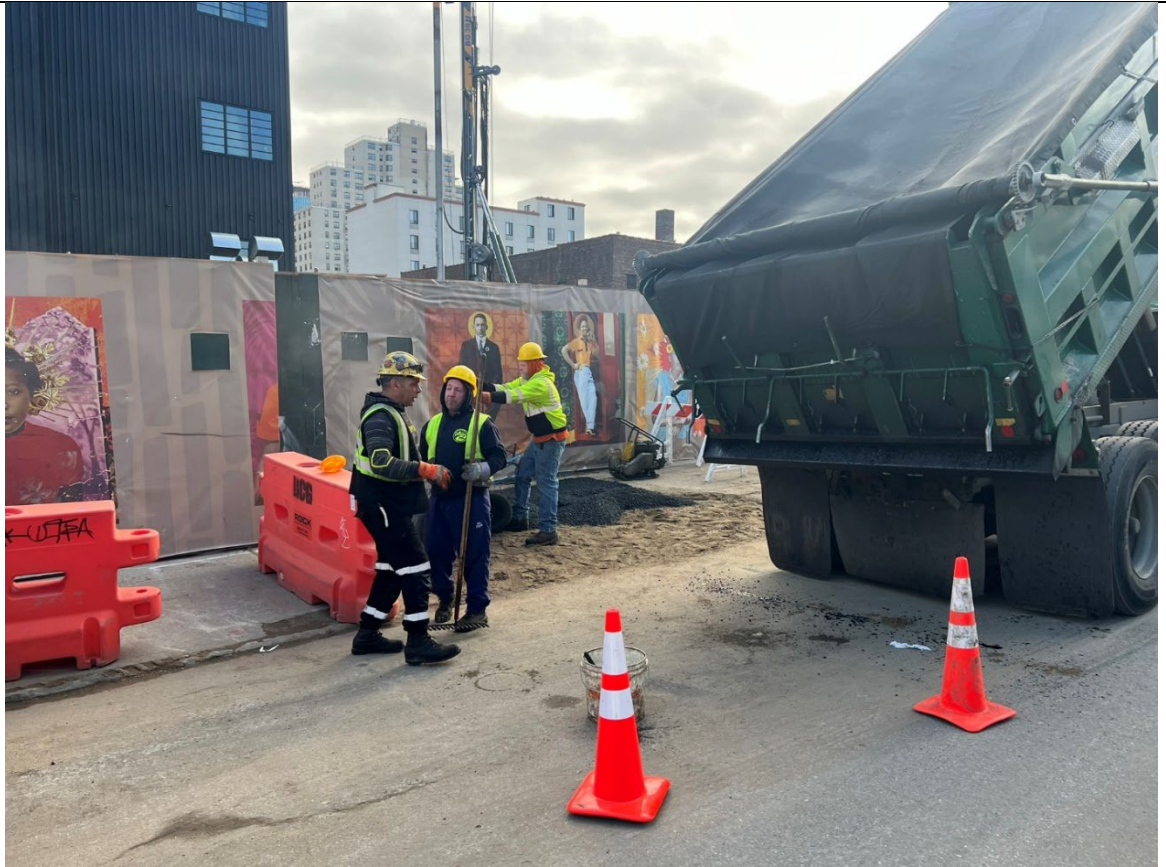
Photo 3- Representative photo of National Grid work adjacent to Douglass Street.
