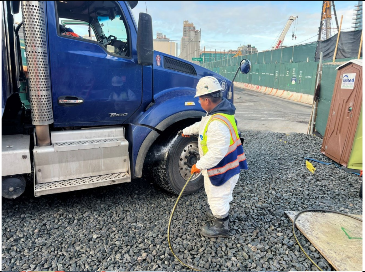
Photo 1- Representative photo of truck tires being washed before leaving the site.
