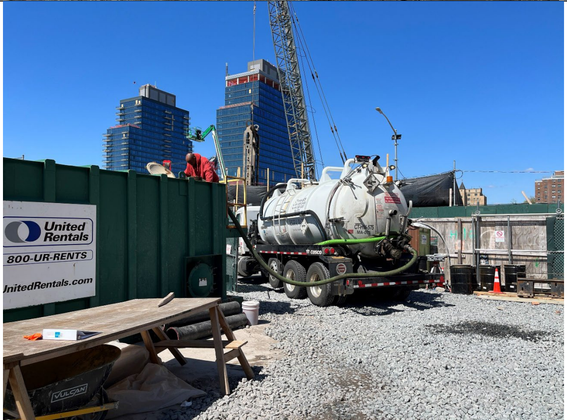
Photo 2- Representative photo of Triumvirate pumping out frac tank.
