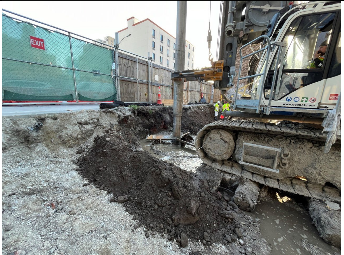
Photo 1- Representative photo of ISS column installation.
