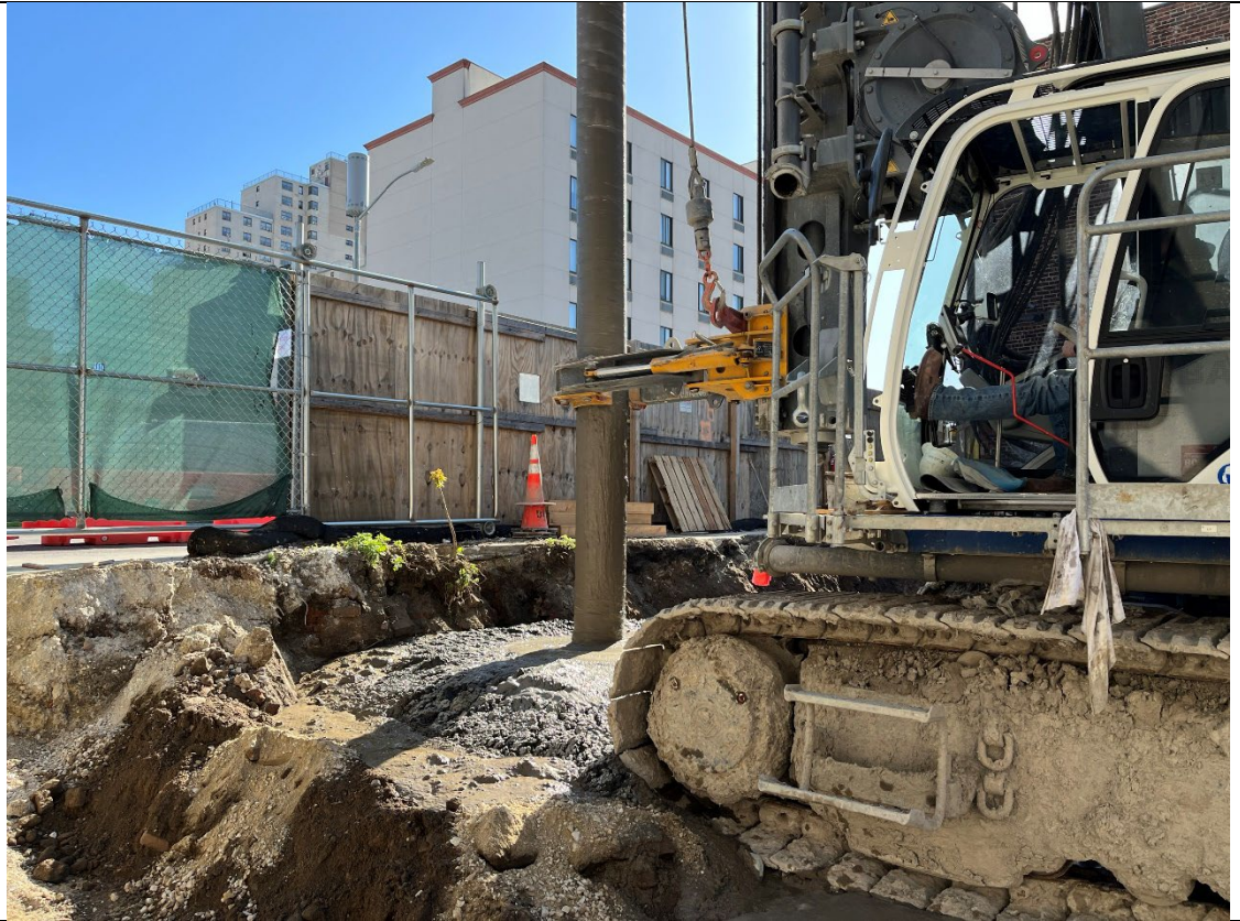
Photo 3- Additional representative photo of ISS column installation.
