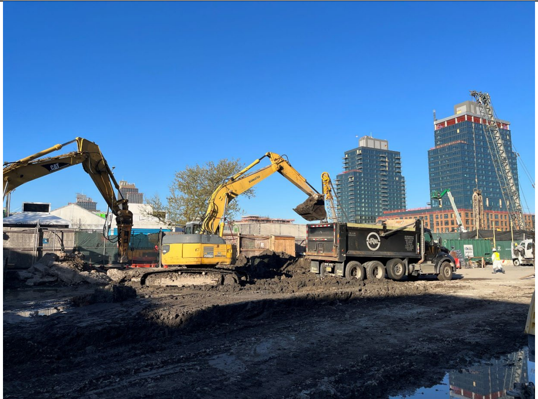
Photo 3- Representative photo of concrete loadout.
