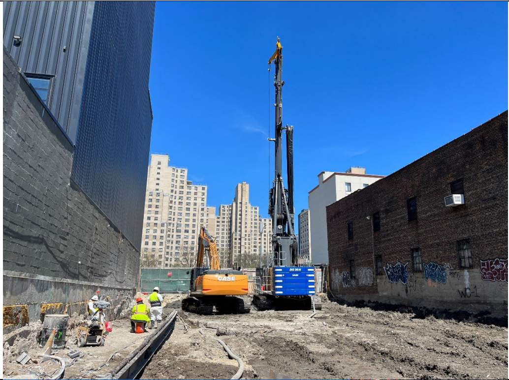
Photo 1- Representative photo of ISS column installation.
