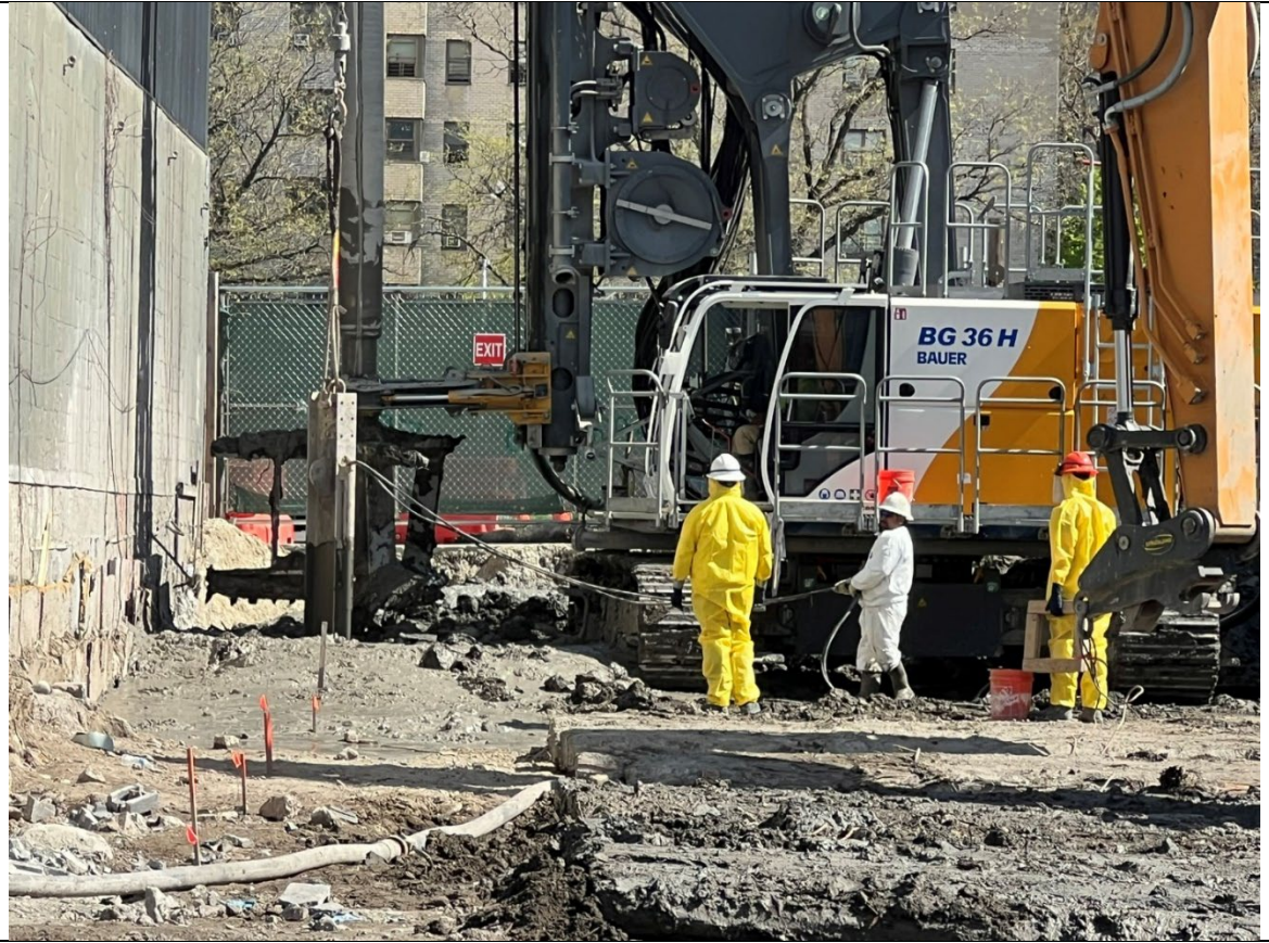
Photo 5- Representative photo of Cascade collecting a wet mix sample.
