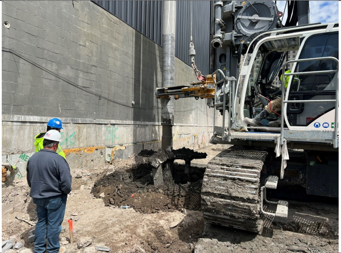
Photo 1- Representative photo of ISS column installation.
