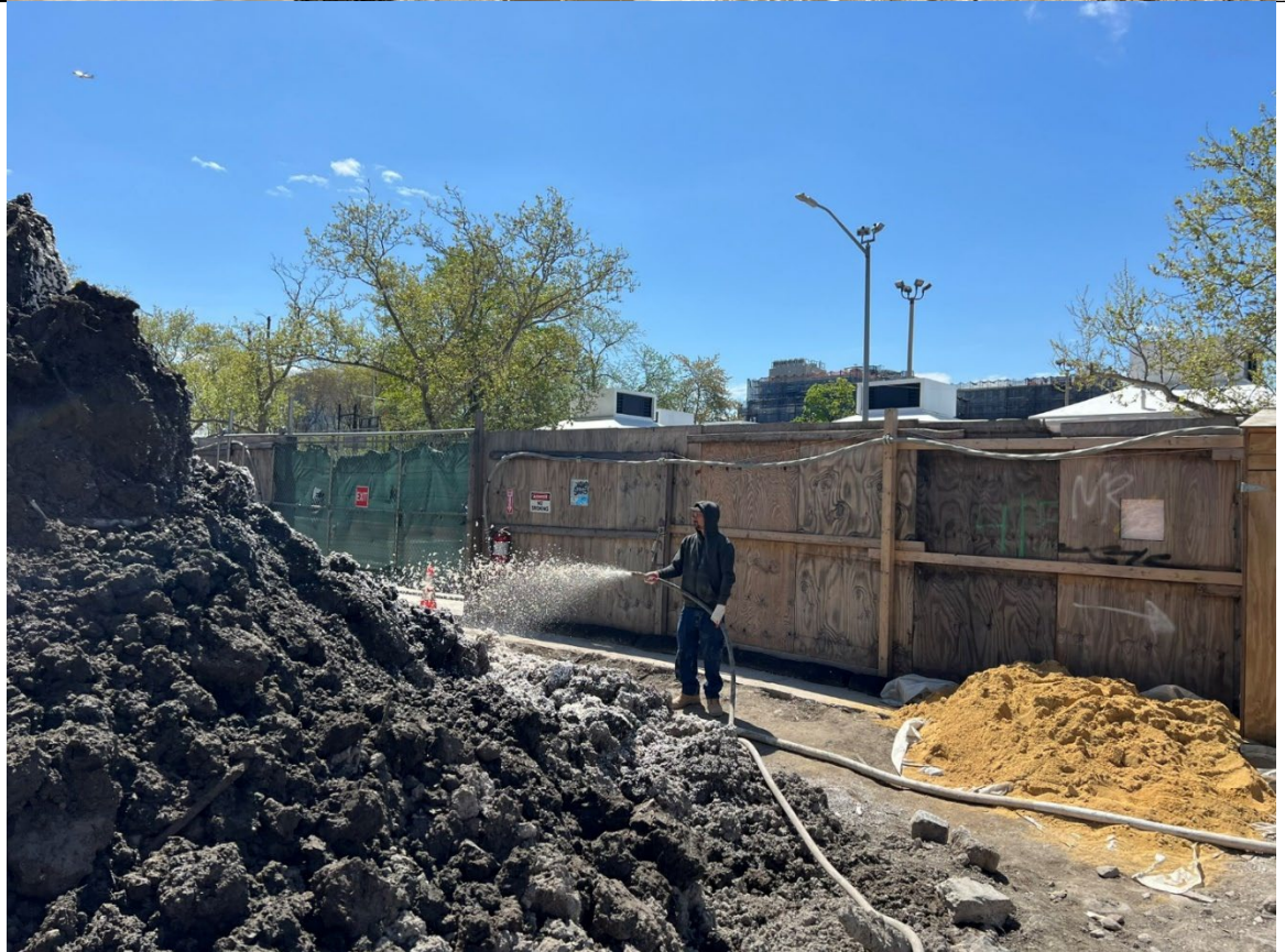
Photo 2- Representative photo of ATMOS foam being sprayed on the stockpile.
