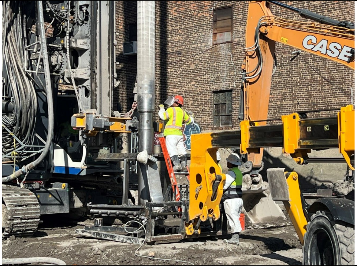
Photo 5- Representative photo of Cascade removing the auger off the rig.
