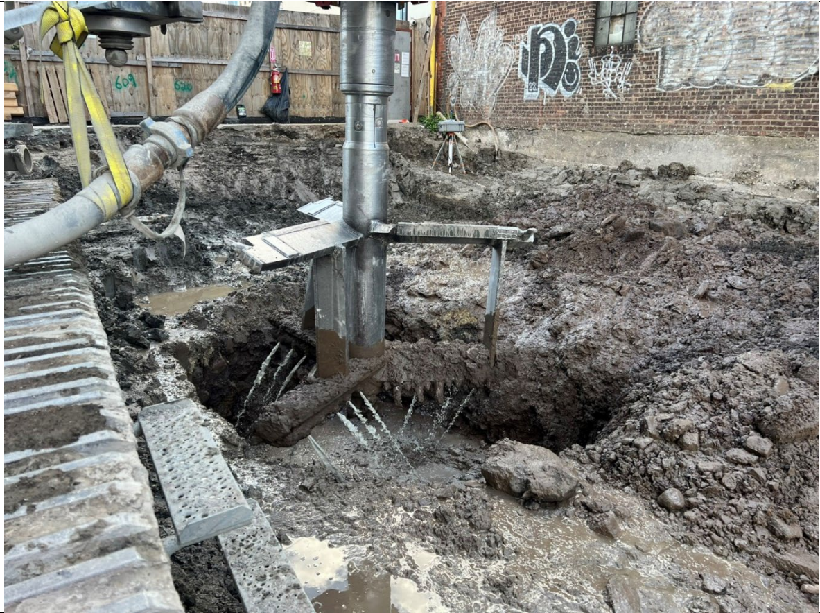
Photo 1- Representative photo of ISS column installation.
