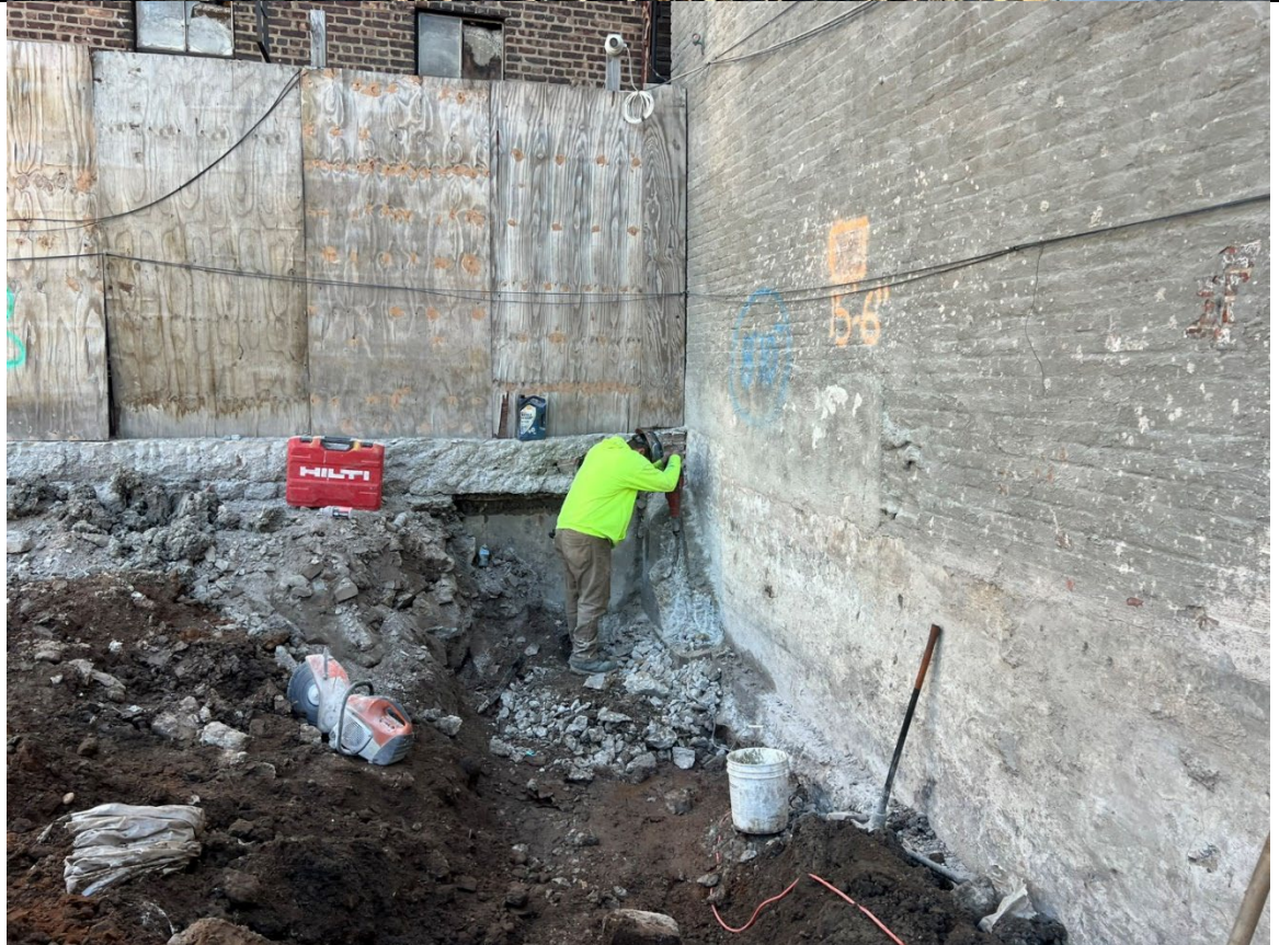
Photo 4- Representative photo of Concrete Courses removing obstructions in the southeast corner of the Site.
