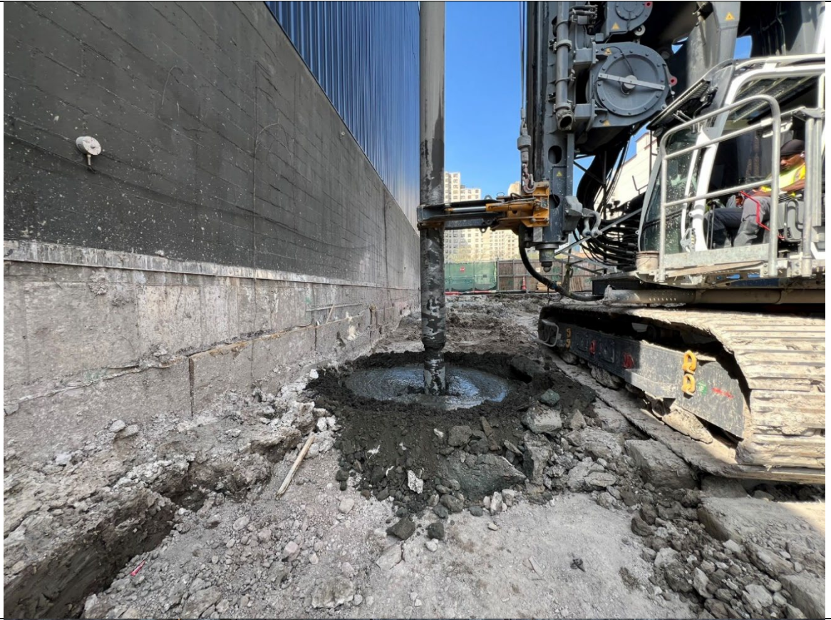
Photo 1- Representative photo of drilling an ISS column.
