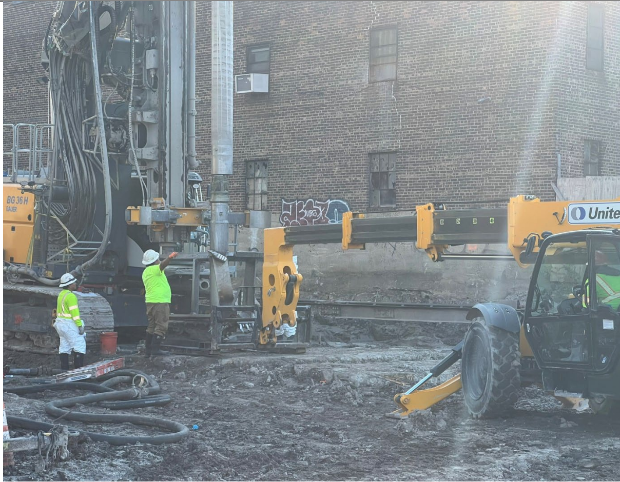
Photo 5- Representative photo of Cascade attaching the auger back on the rig.
