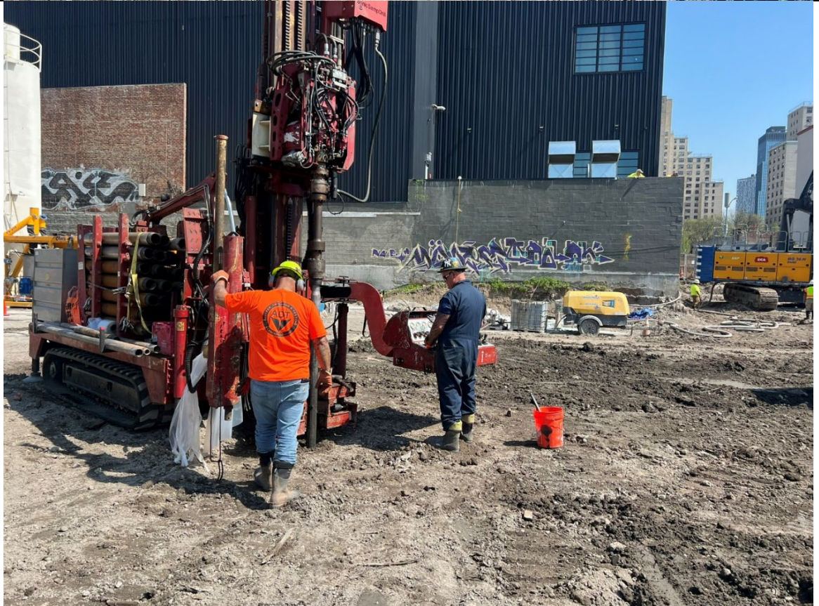
Photo 4- Representative photo of ADT performing QA/QC coring.
