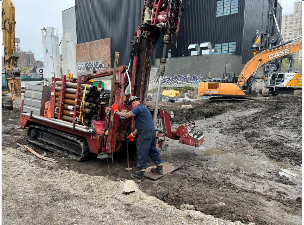
Photo 4- Representative photo of ADT during QA/QC coring.
