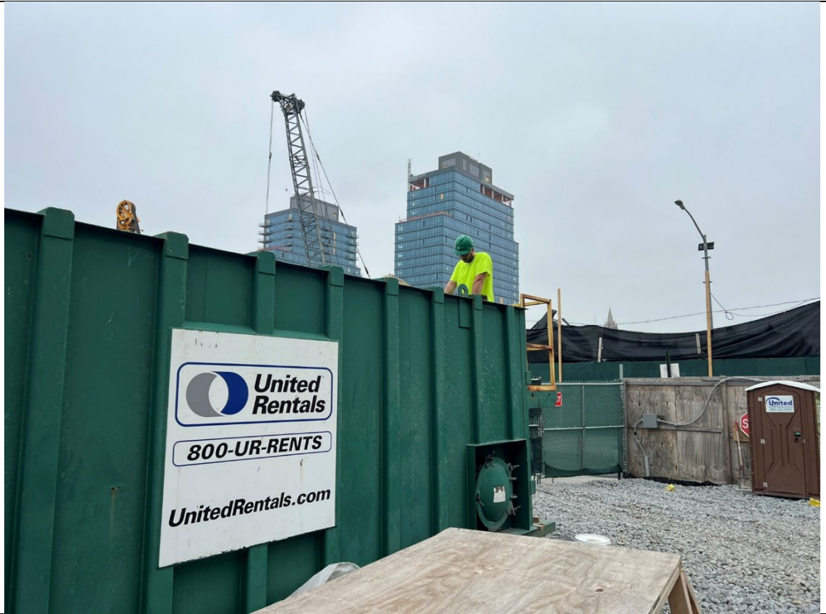
Photo 3- Representative photo of Triumvirate removing water from the frac tank.
