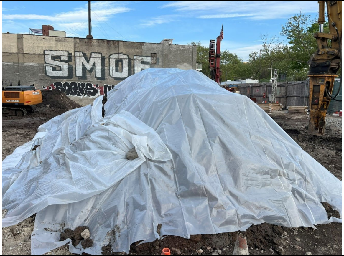
Photo 5- Representative photo of a stockpile covered at the end of the day.
