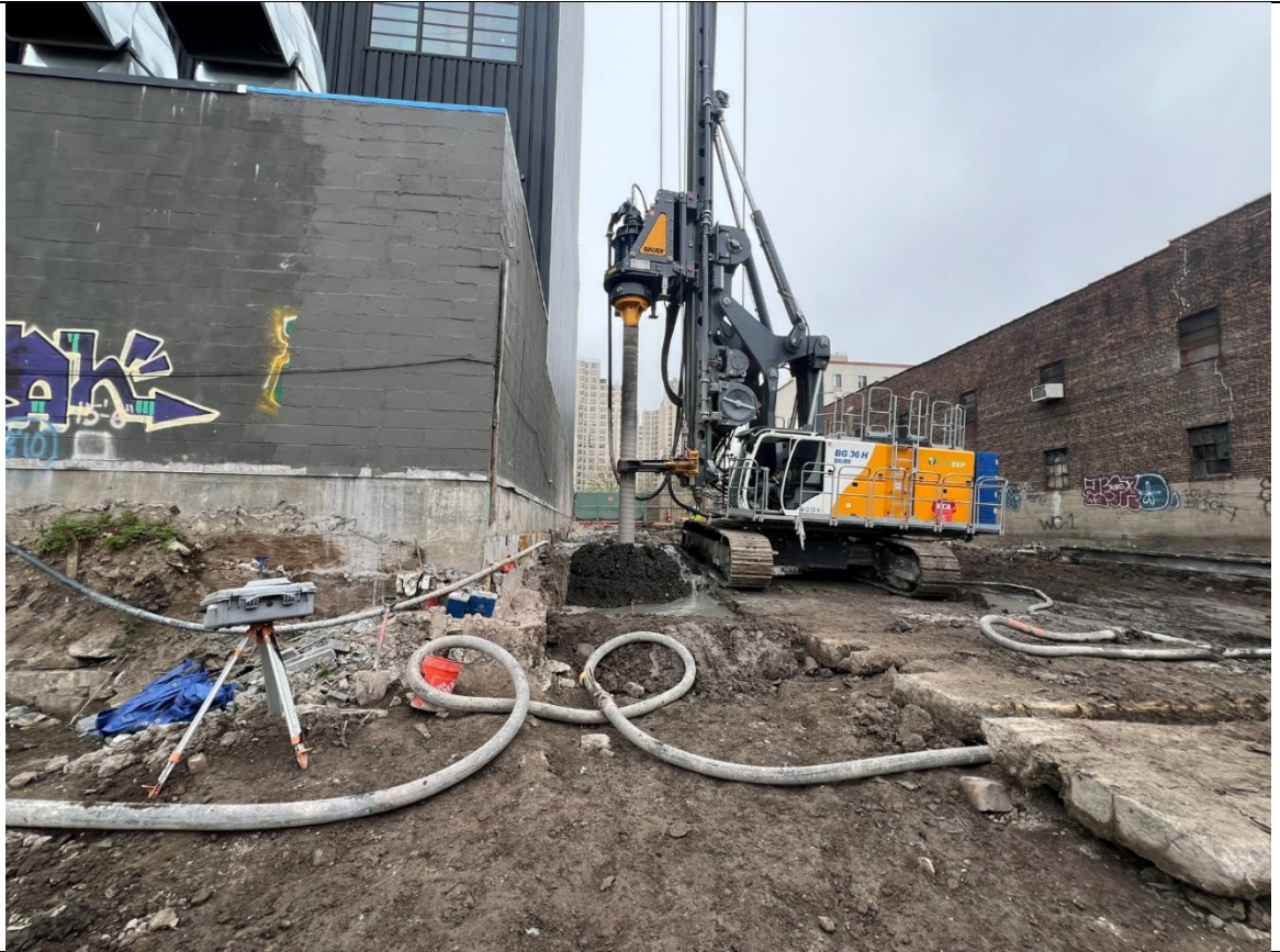
Photo 1- Representative photo of drilling an ISS column.
