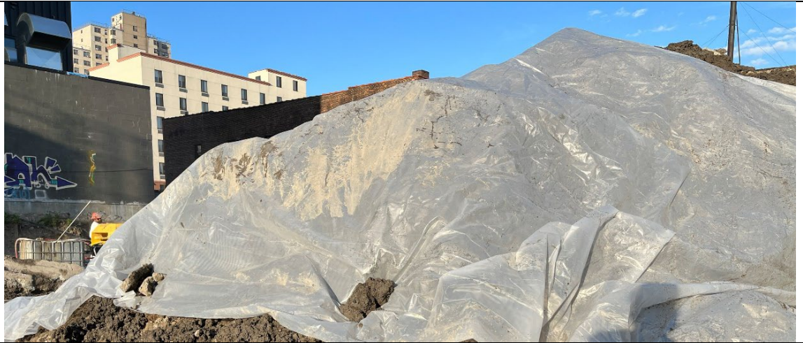
Photo 5- Representative photo of a stockpile covered at the end of the day.
