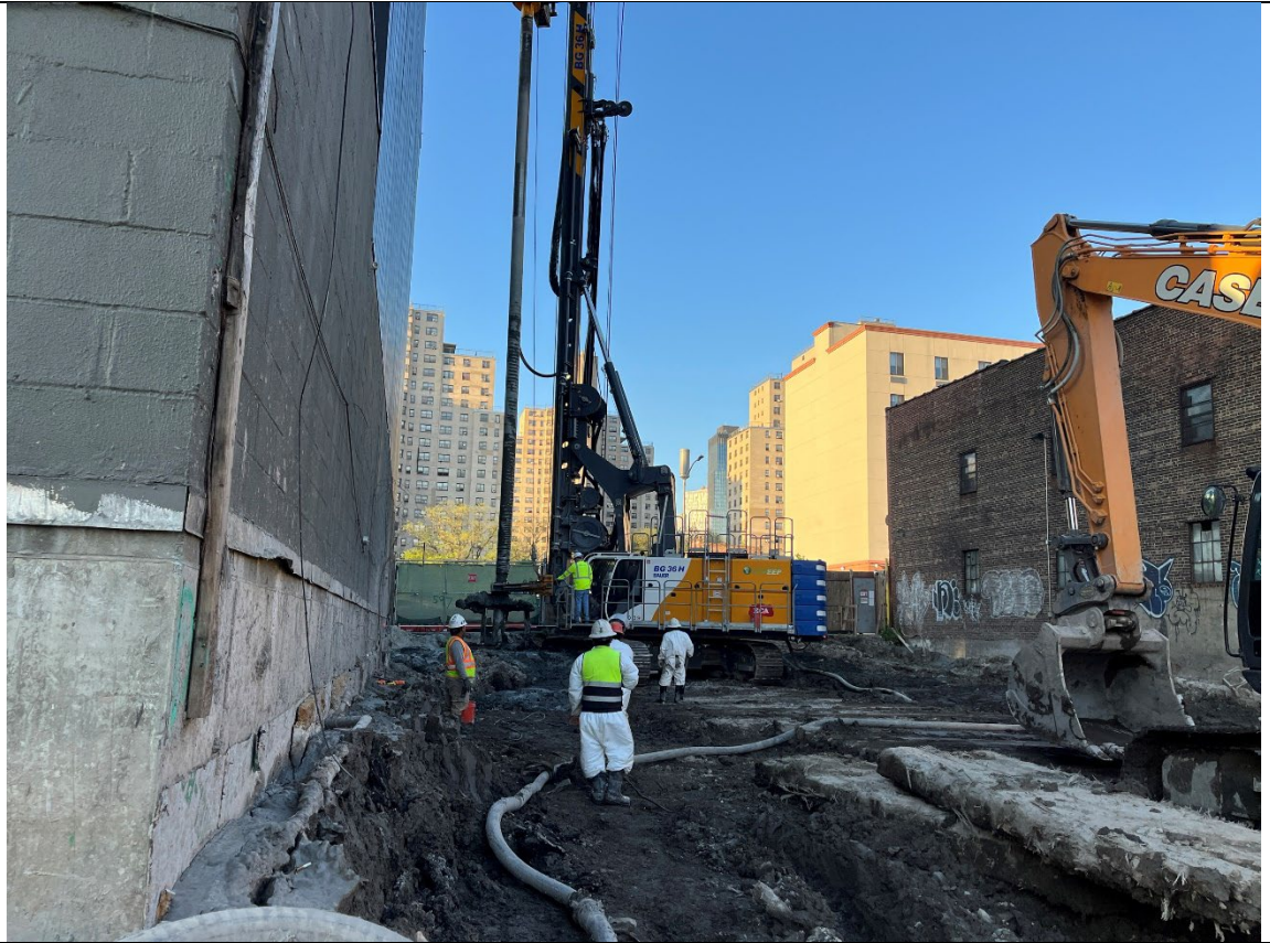
Photo 3- Representative photo of auger paused during column 630 downstroke 1.
