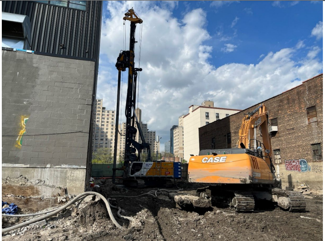
Photo 1- Representative photo of drilling an ISS column.
