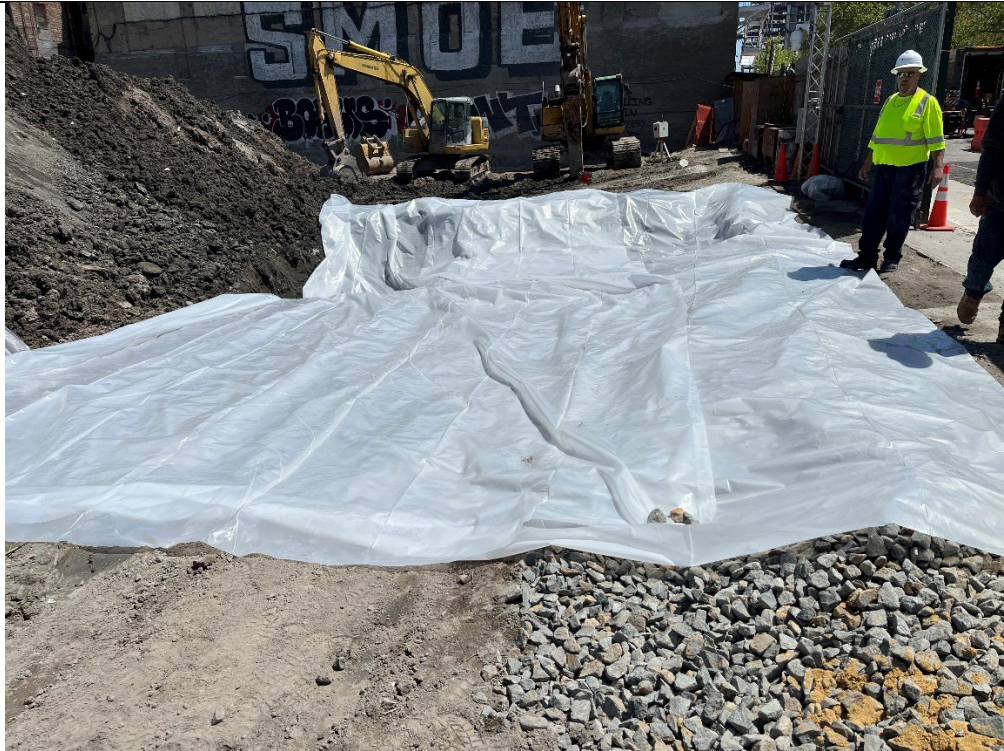
Photo 1- Representative photo of plastic lining for new truck pad.
