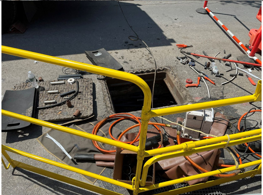
Photo 4- Representative photo of Con Edison work on Douglass Street.
