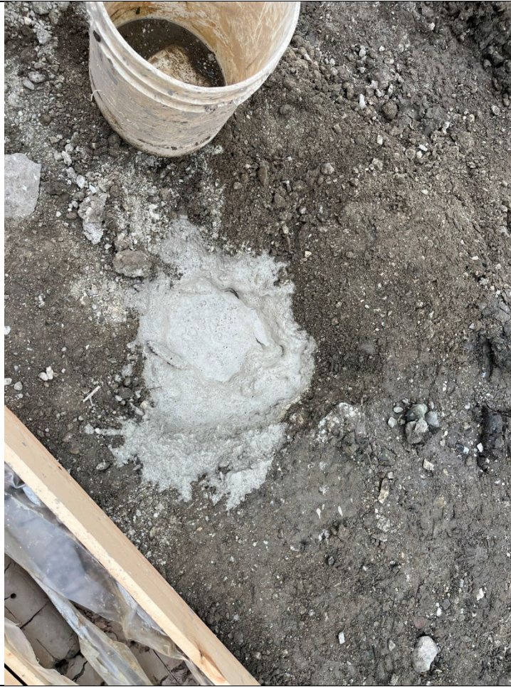
Photo 5- Representative photo of a grouted coring hole.
