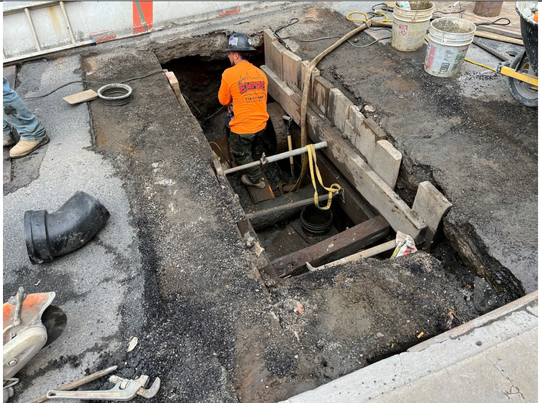
Photo 3- Representative photo of Empire work on sewer connection.
