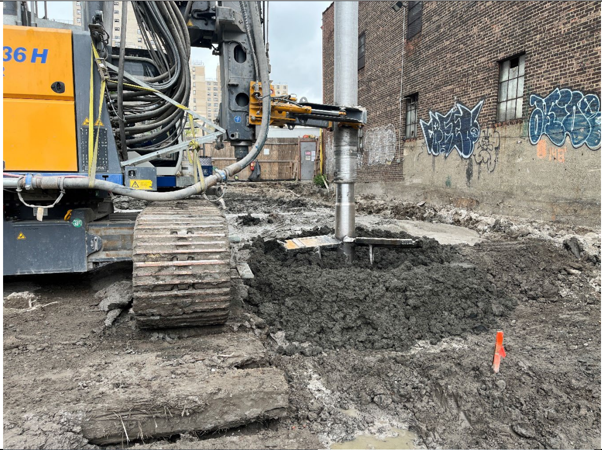
Photo 3- Representative photo of ISS column installation.
