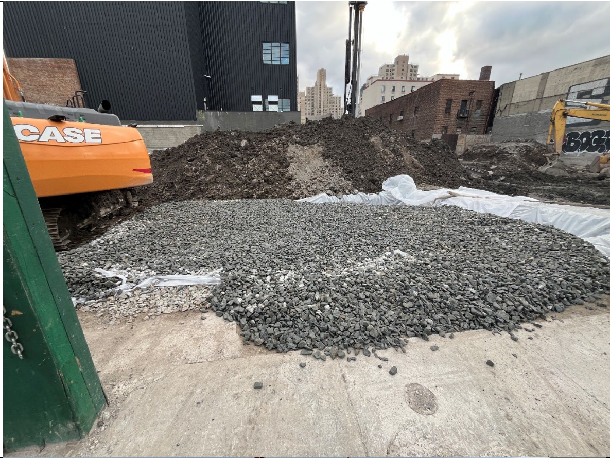
Photo 1- Representative photo of new truck pad.
