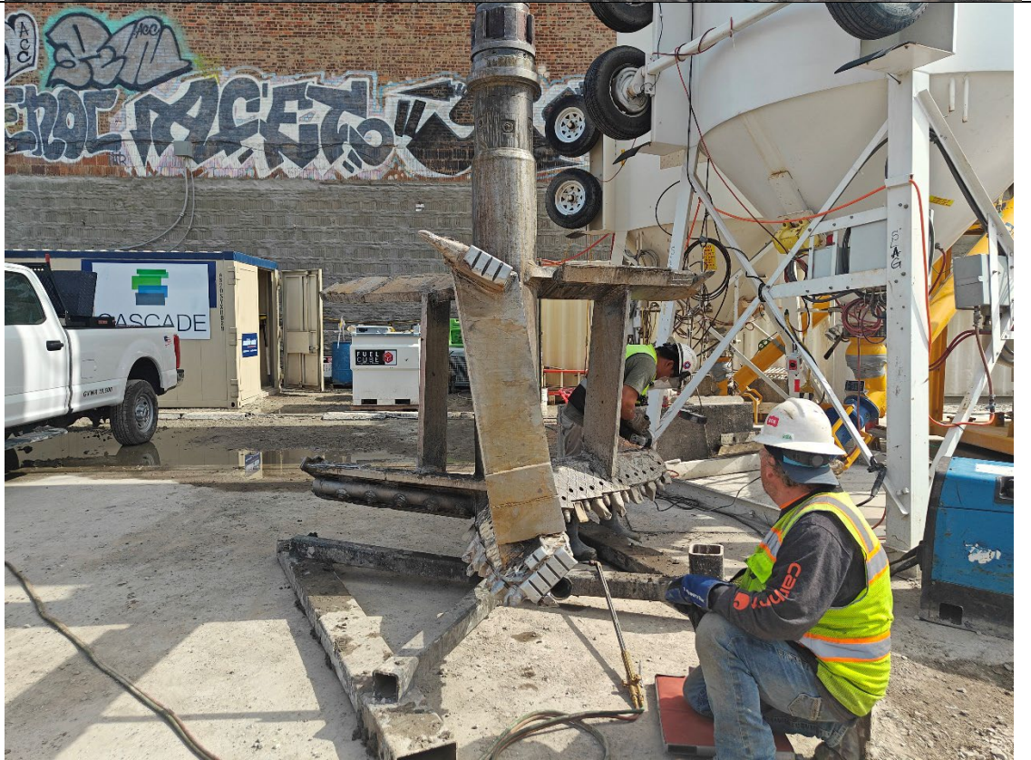
Photo 2- Representative photo of rig maintenance.
