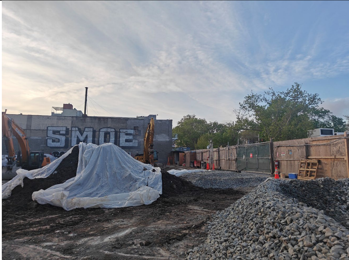
Photo 4- Representative photo of the Site nearing the end of days activities.
