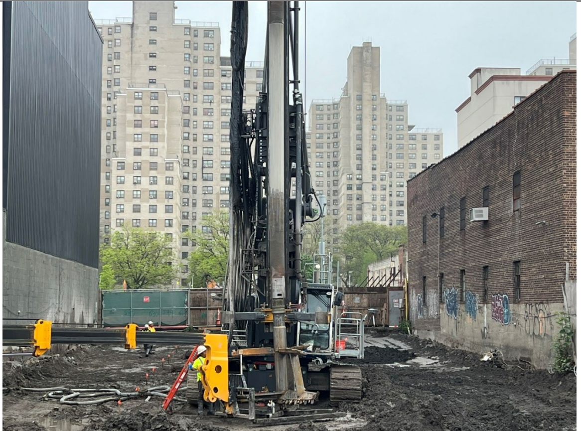
Photo 1- Representative photo of Cascade attaching the auger to the rig.
