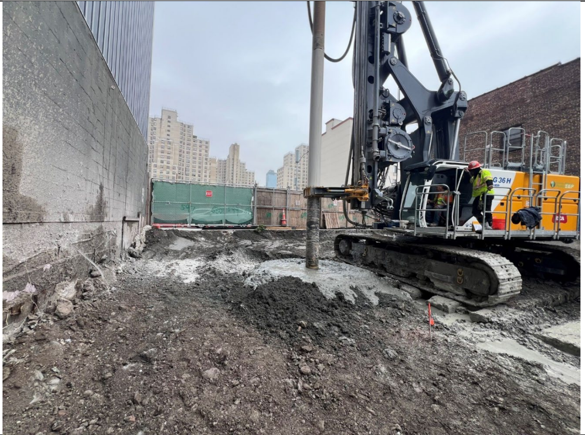
Photo 3- Representative photo of ISS column installation.
