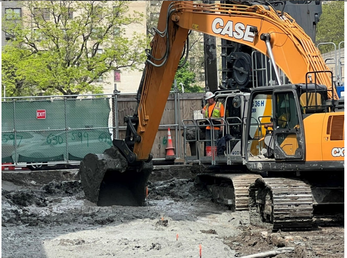
Photo 2- Representative photo of cascade removing a shallow obstruction.
