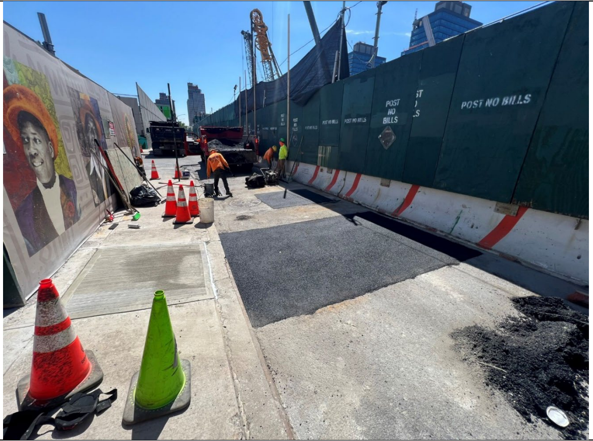
Photo 5- Representative photo of completed work along Nevins Street by Empire.
