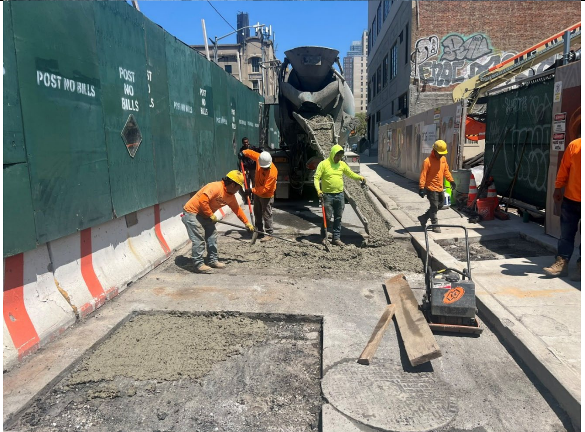
Photo 4- Representative photo of work along Nevins Street by Empire.
