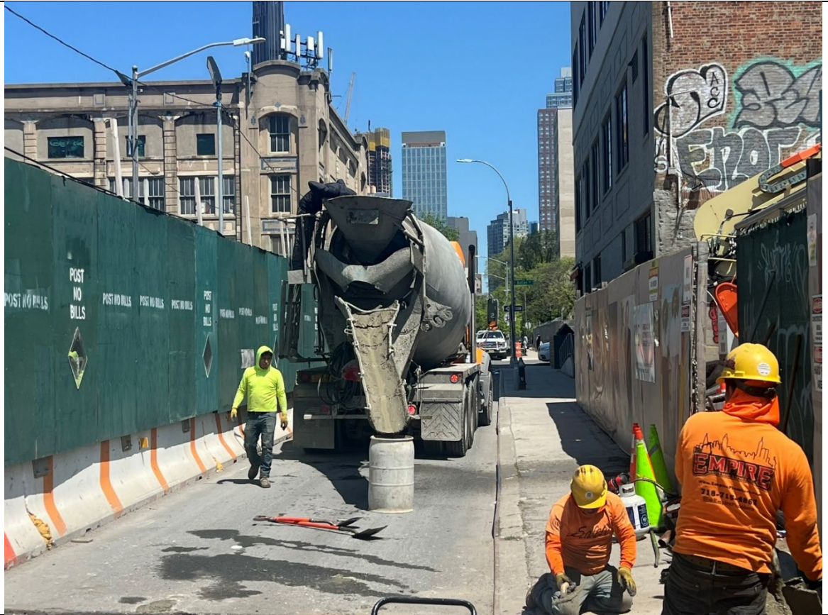
Photo 1- Representative photo of washout being put into a drum.
