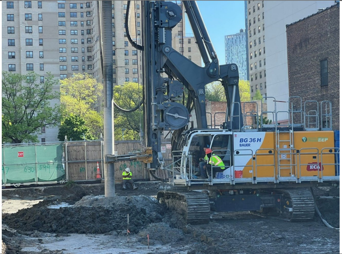
Photo 3- Representative photo of ISS column installation.
