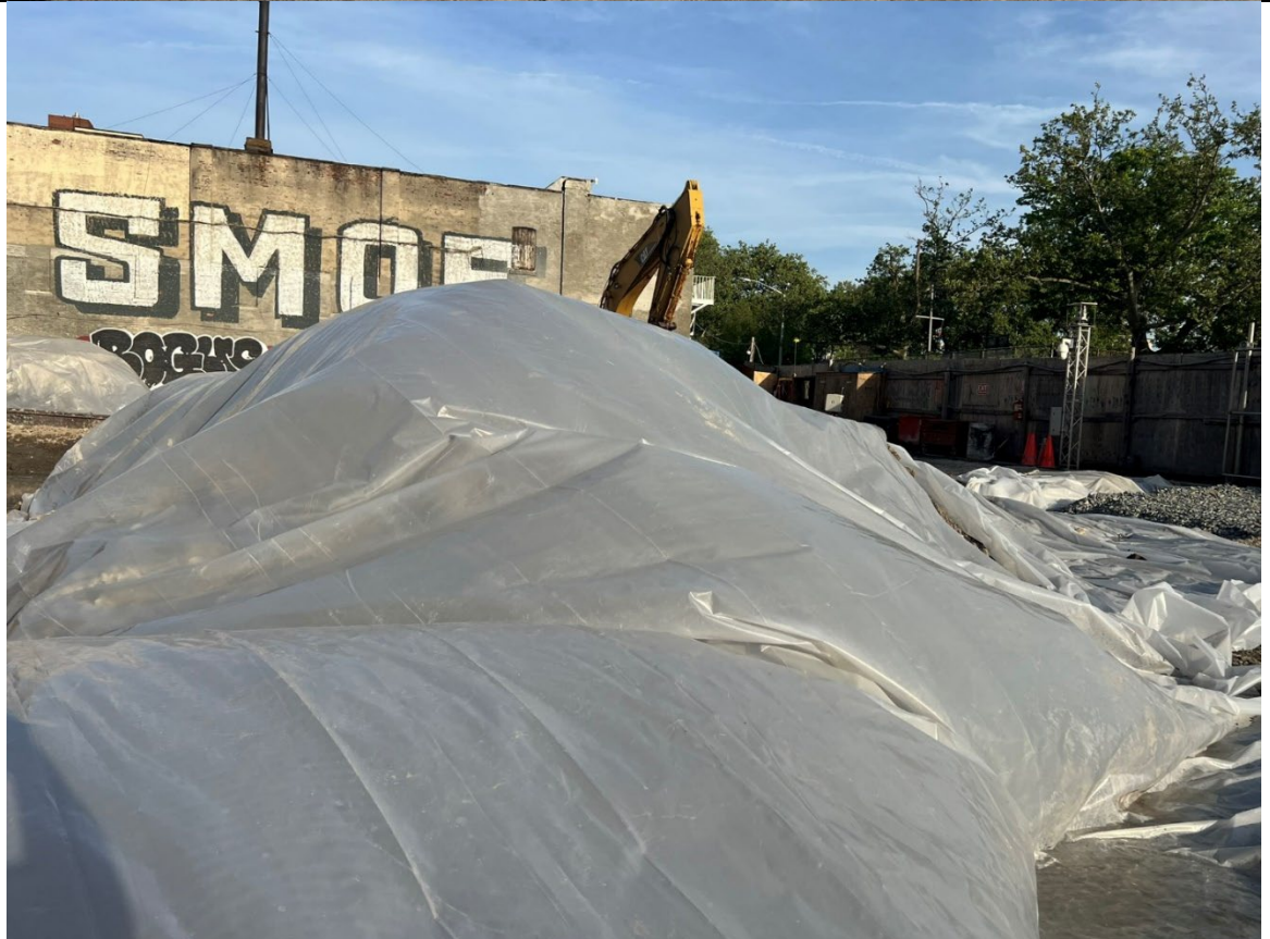
Photo 2- Representative photo of swell stockpile covered at the end of the day.
