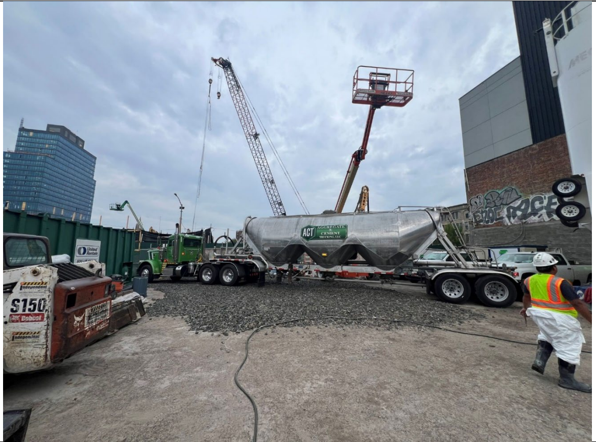
Photo 1- Representative photo of a slag delivery.
