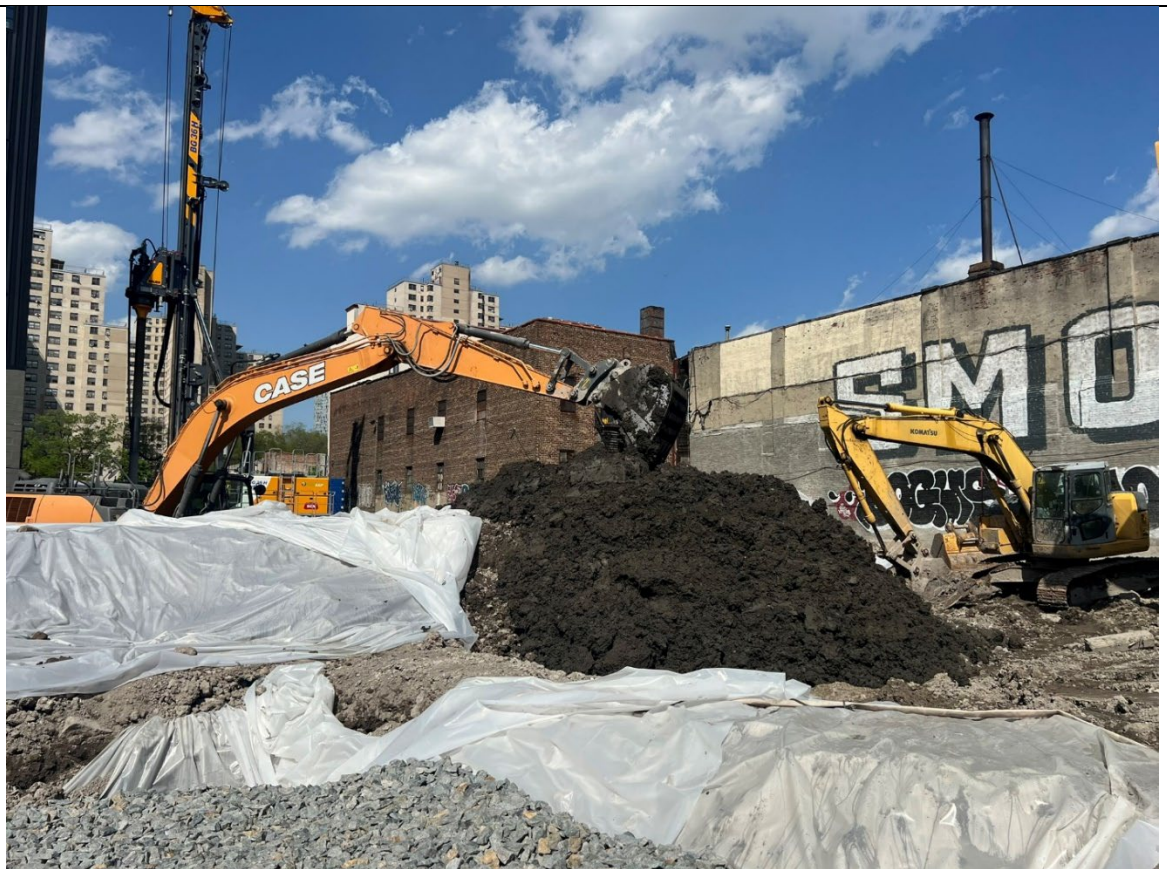
Photo 4- Representative photo of stockpiling ISS swell material.
