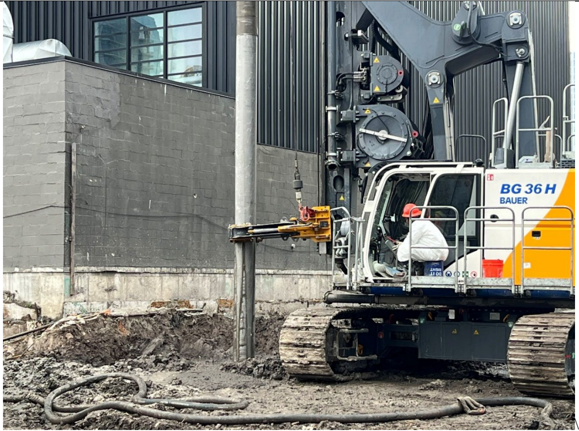
Photo 3- Representative photo of ISS column installation.
