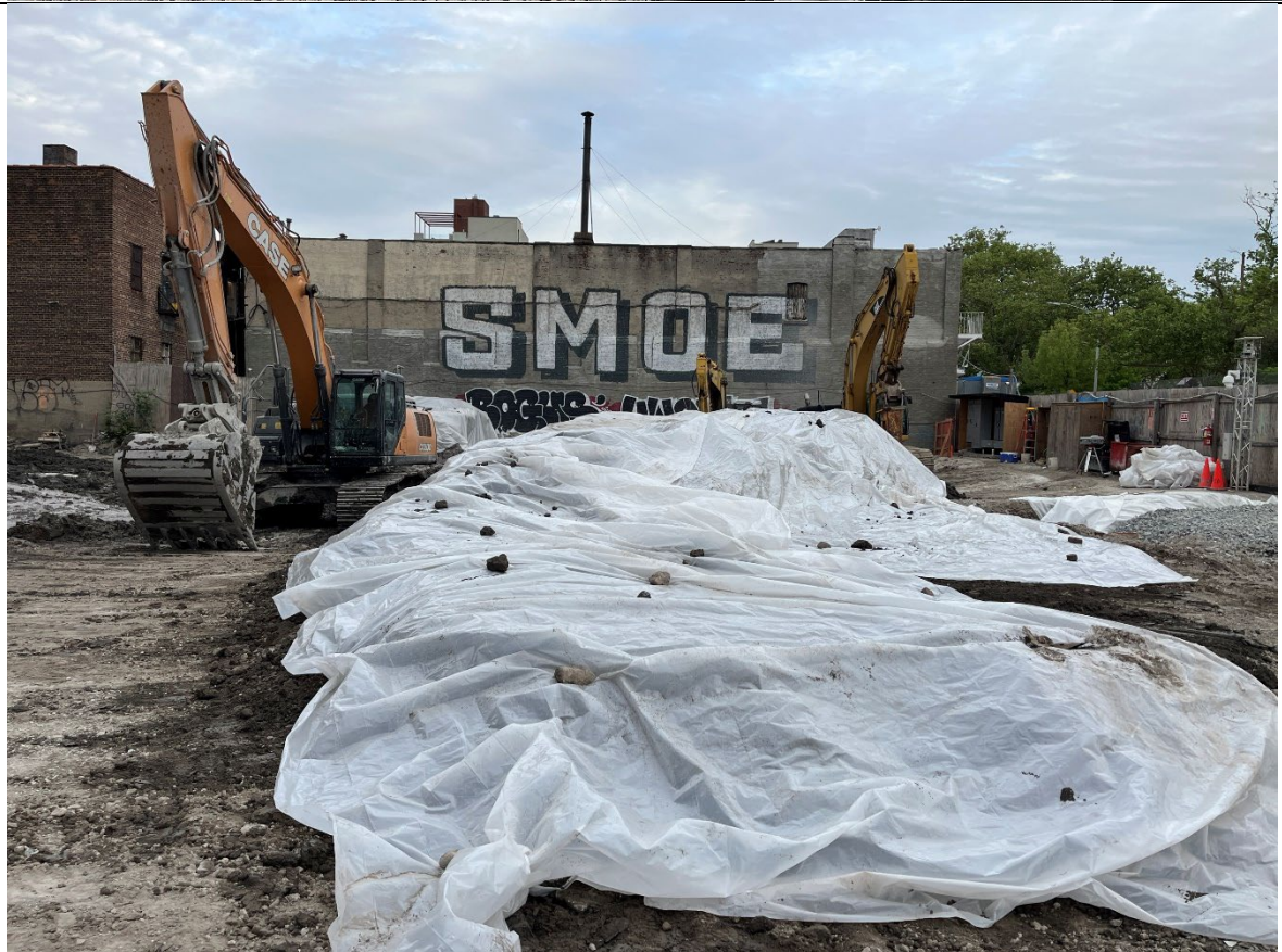
Photo 2- Representative photo of swell stockpile covered at the end of the day.
