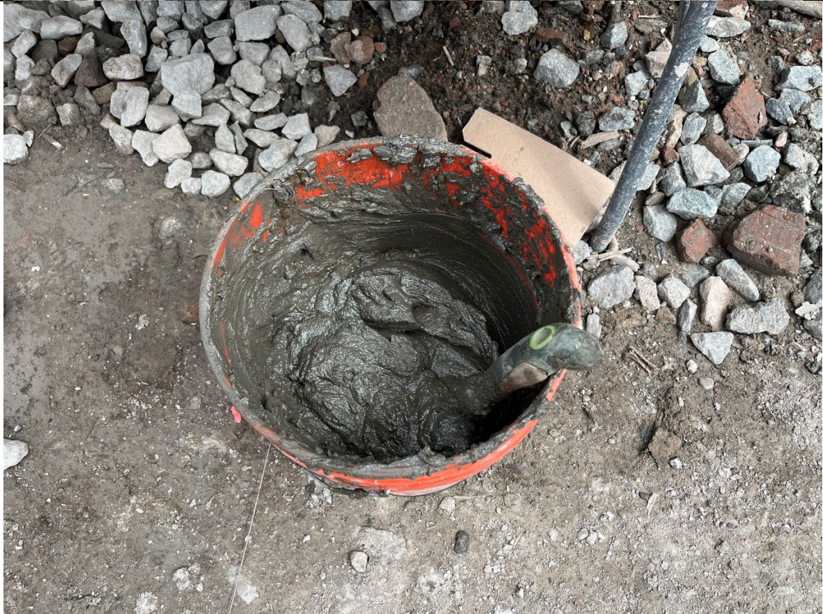
Photo 4- Representative photo of wet mix sample collected from Column 531.
