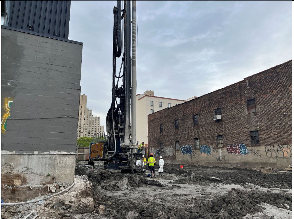
Photo 3- Representative photo of auger teeth replacement.
