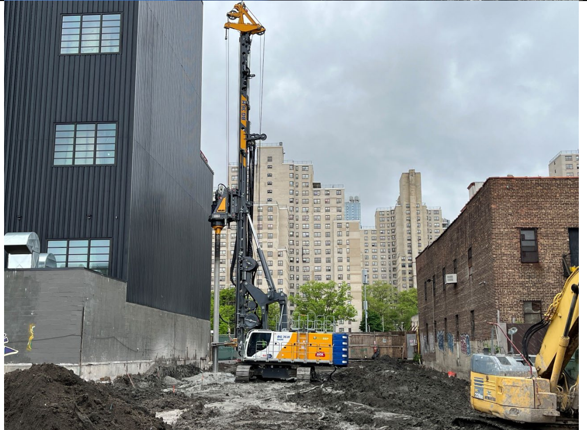
Photo 2- Representative photo of ISS column installation.
