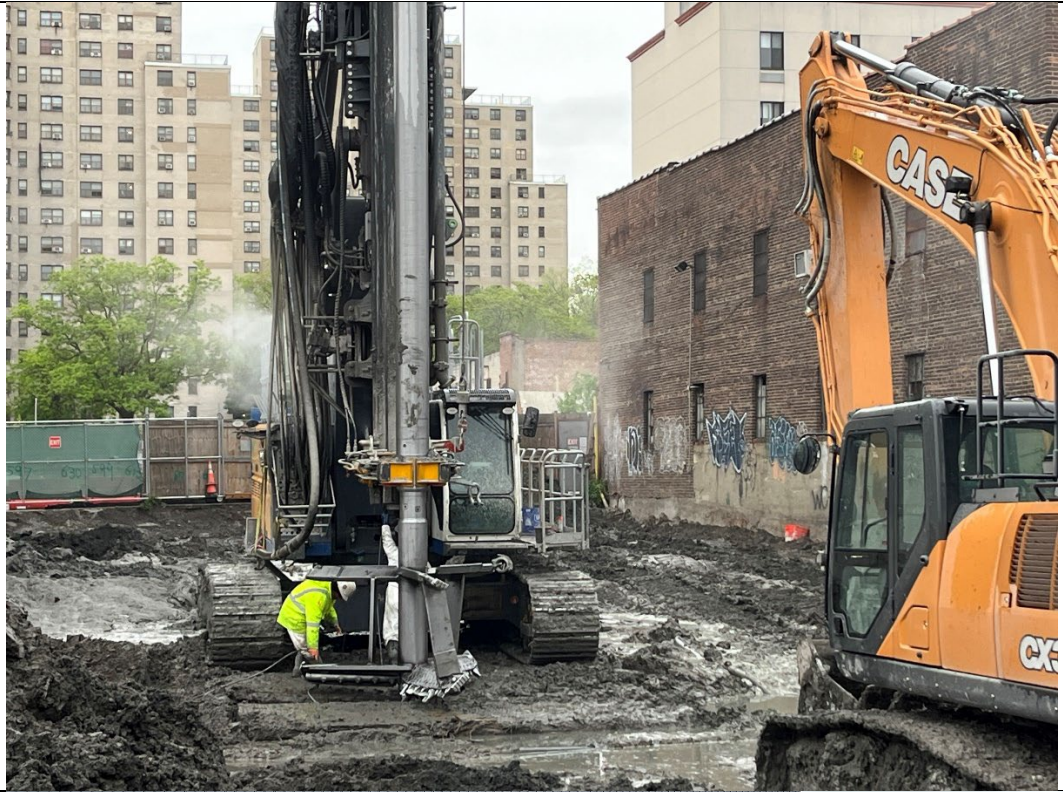
Photo 3- Representative photo of auger maintenance and decontamination.
