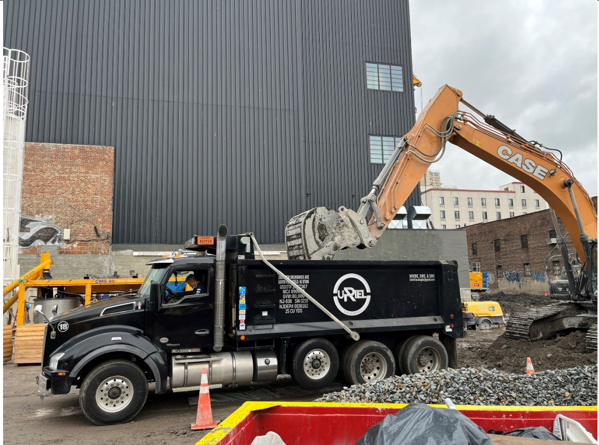
Photo 4- Representative photo of swell material load out.
