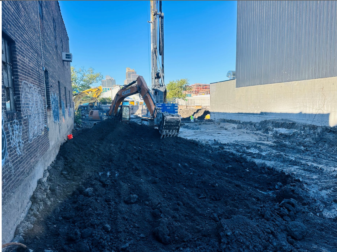
Photo 4- Representative photo of stockpiling ISS swell material.
