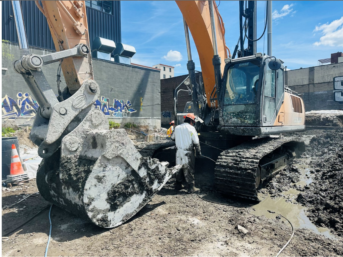
Photo 3- Representative photo of excavator being washed.
