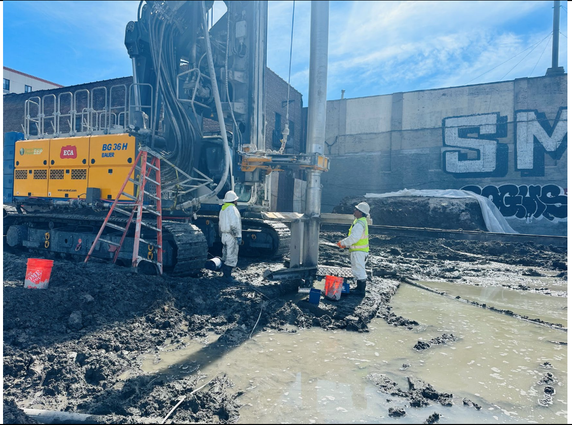
Photo 2- Representative photo of rig maintenance.
