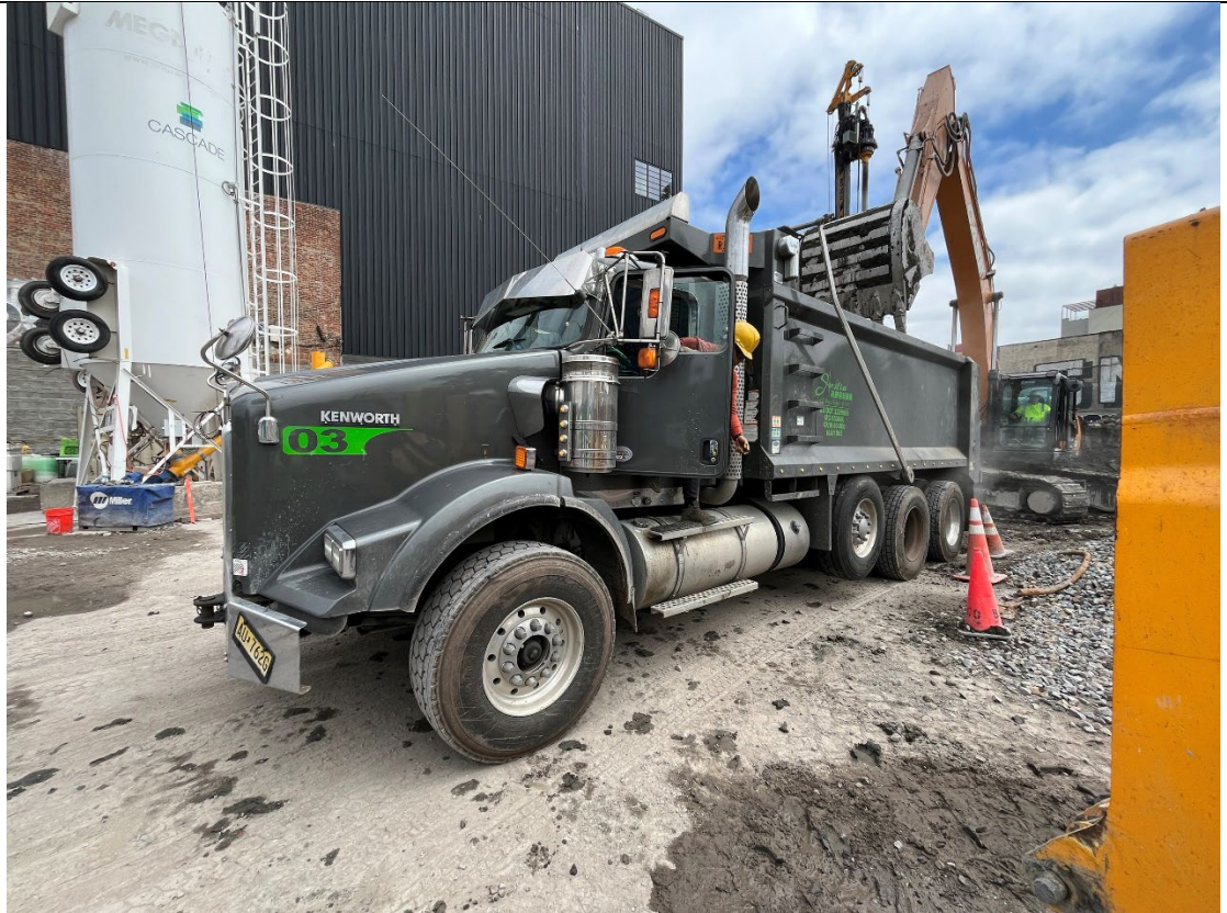
Photo 1- Representative photo of swell material trucking for offsite disposal.
