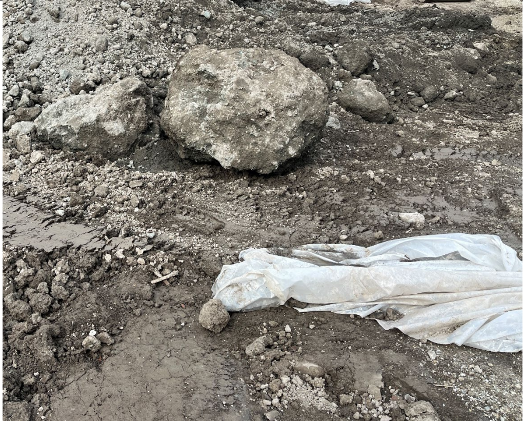
Photo 4- Representative photo of obstructions removed from northern alley.
