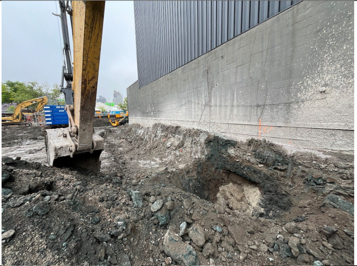
Photo 3- Representative photo of Cascade excavating for obstructions.
