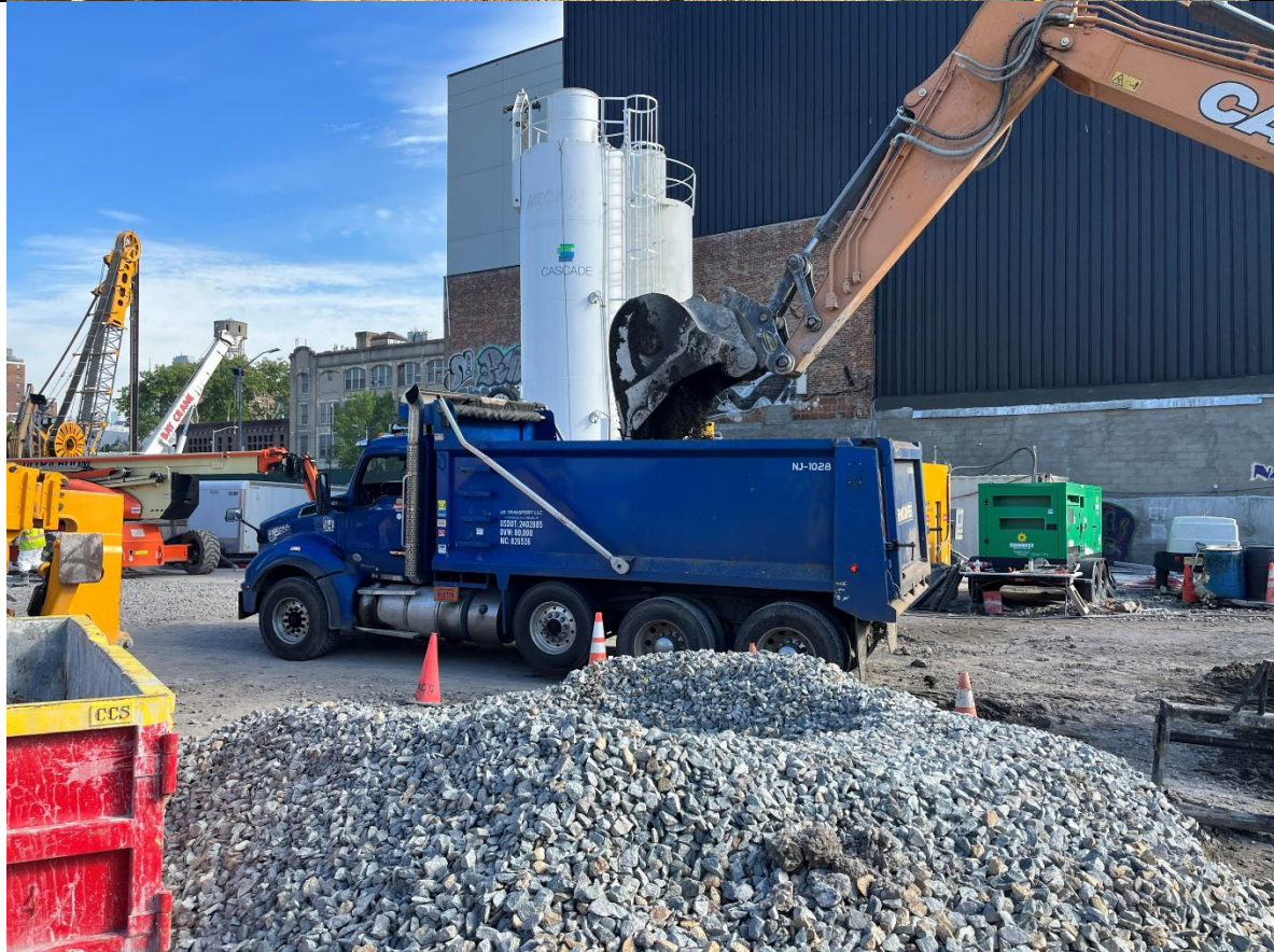
Photo 4- Representative photo of swell material load out.
