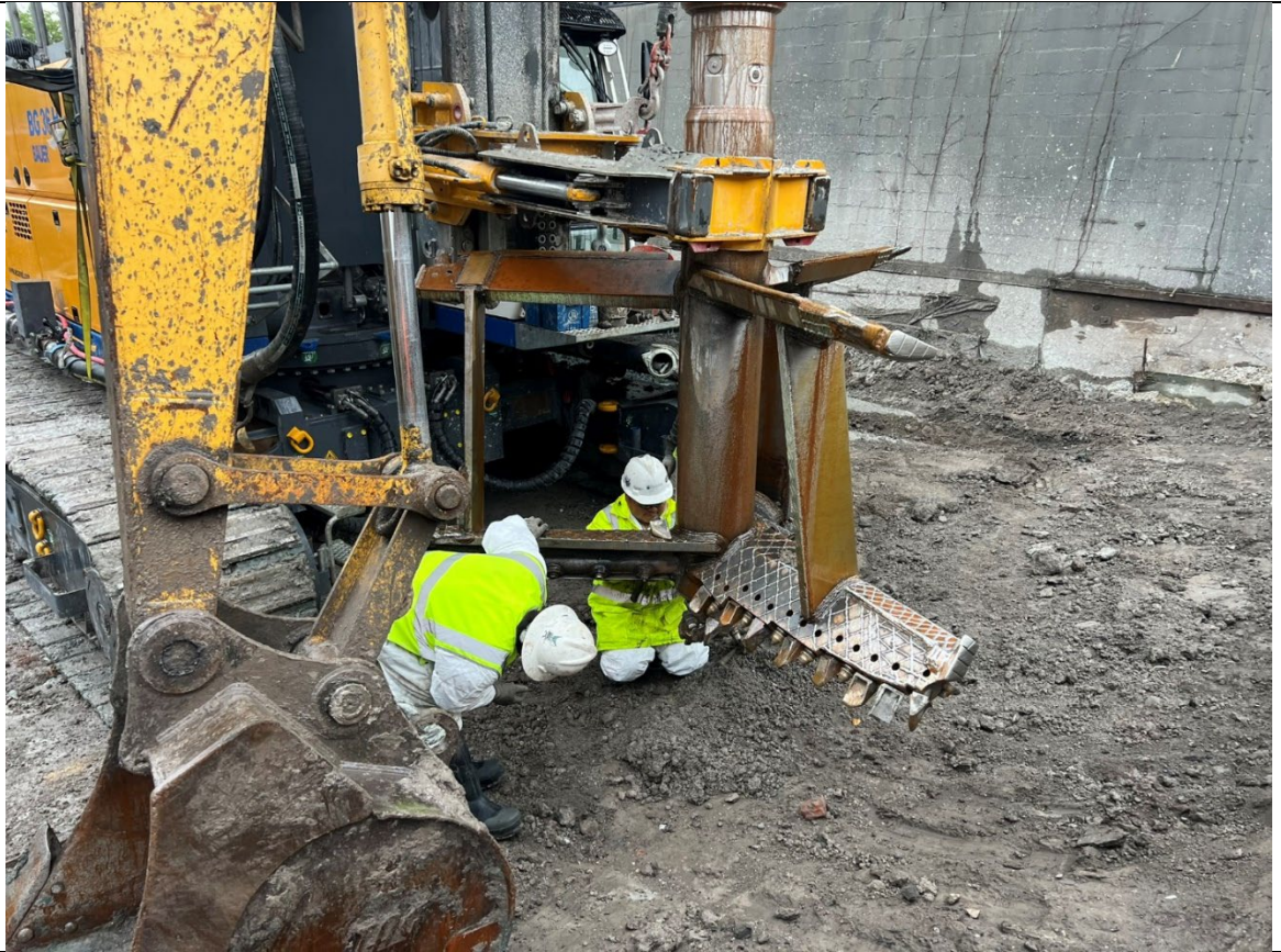
Photo 3- Representative photo of new teeth being put on the auger.
