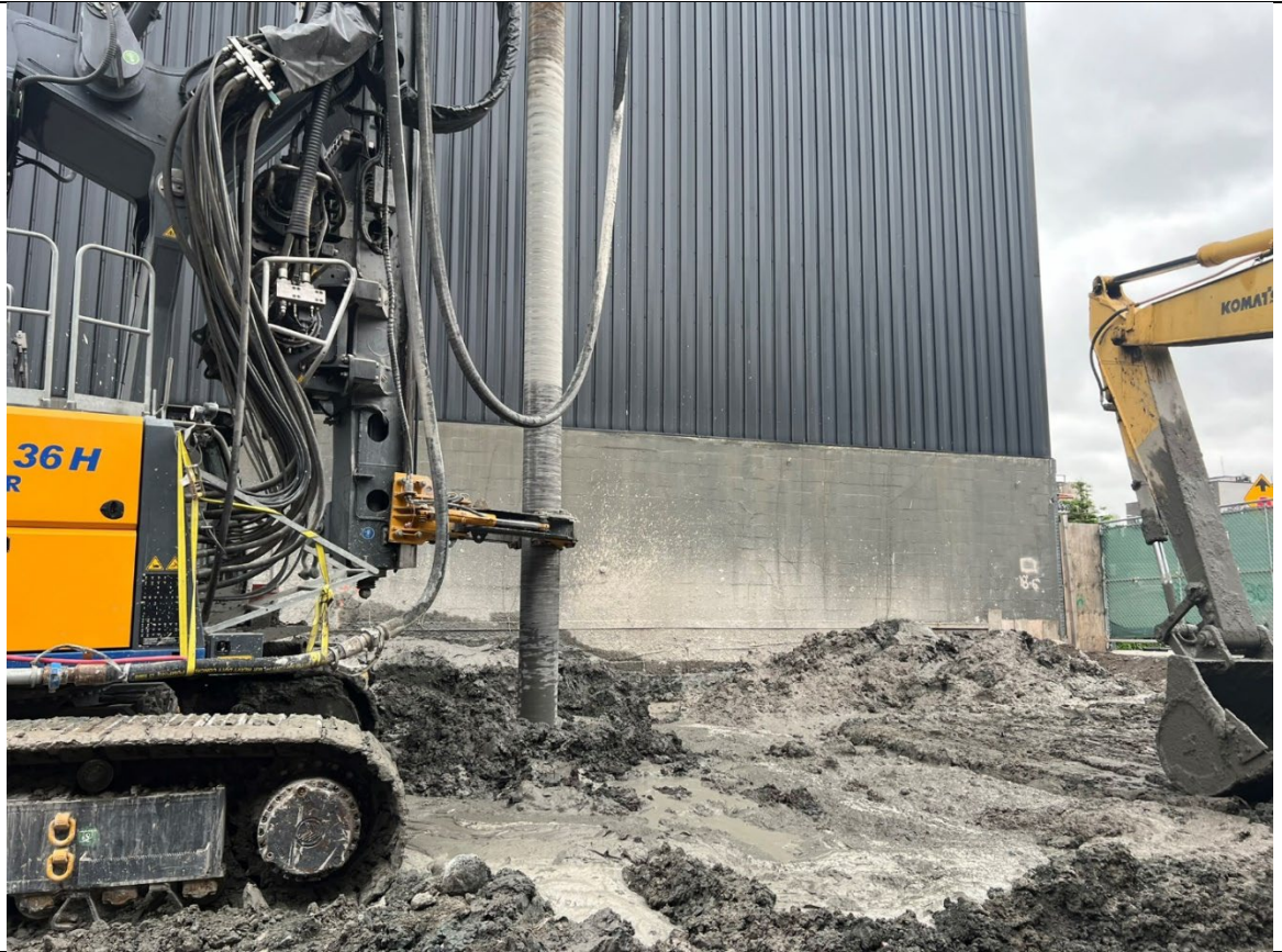
Photo 1- Representative photo of ISS column installation.
