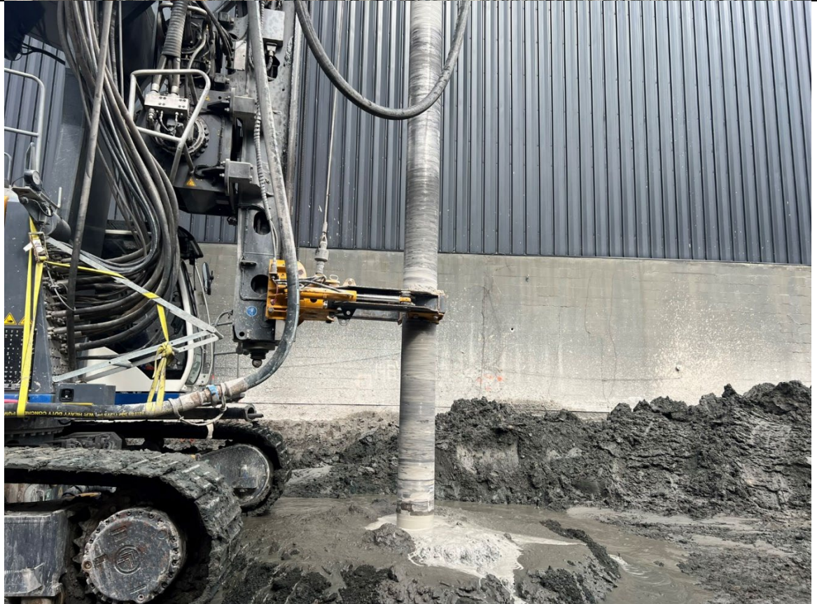
Photo 4- Representative photo of ISS column being drilled.
