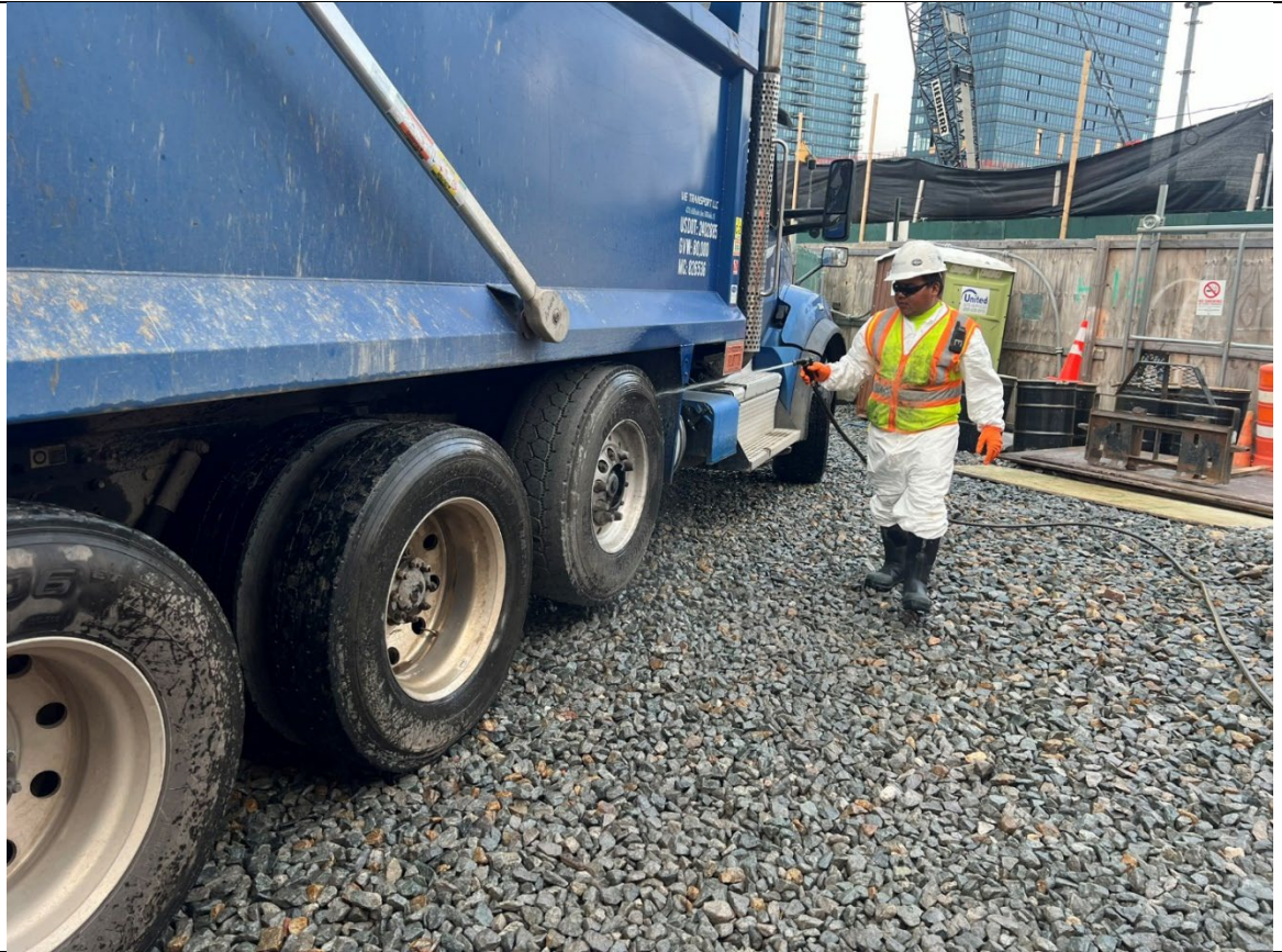
Photo 3- Representative photo of tires being washed.
