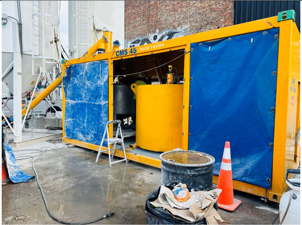
Photo 3- Representative photo of grout mixing machine being washed and serviced.
