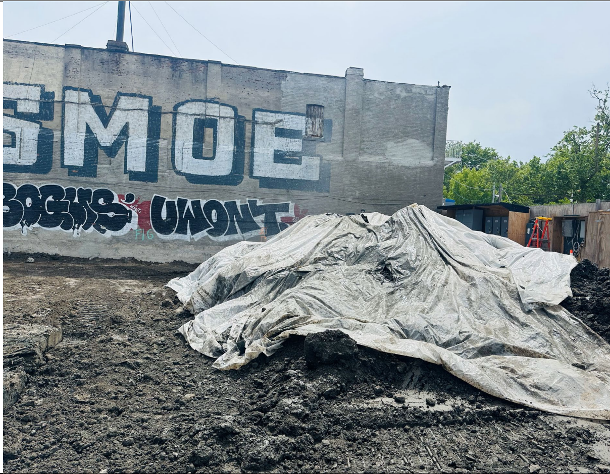
Photo 4- Representative photo of stockpile ISS swell material being covered with plastic.
