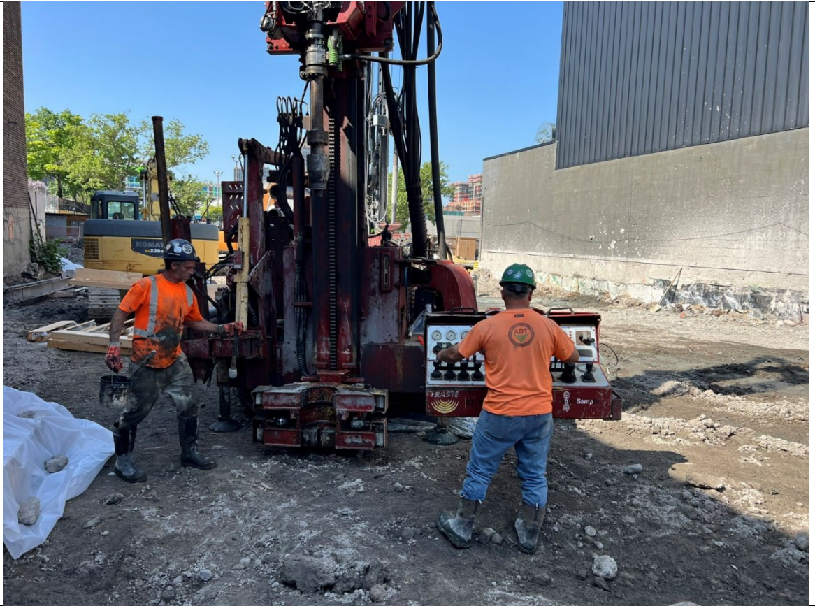
Photo 3- Representative photo of drillers drilling a QA/QC core.
