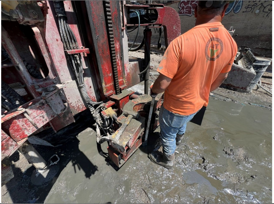
Photo 5- Representative photo of ADT grouting a QA/QC coring location.
