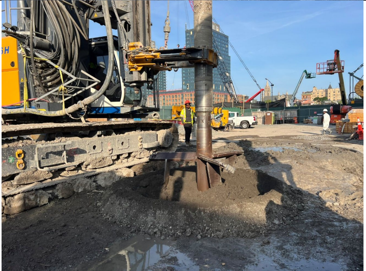
Photo 4- Representative photo of ISS column being drilled.
