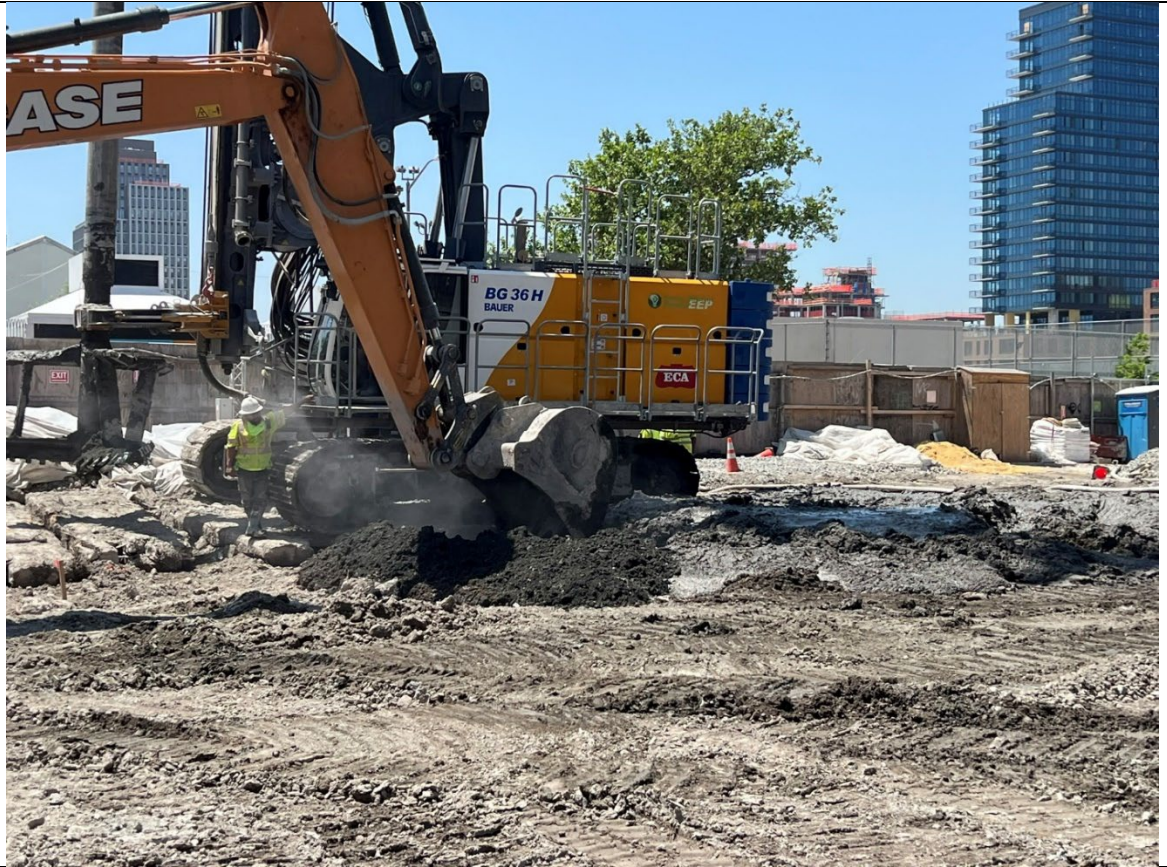
Photo 1- Representative photo of removing a shallow obstruction from column.
