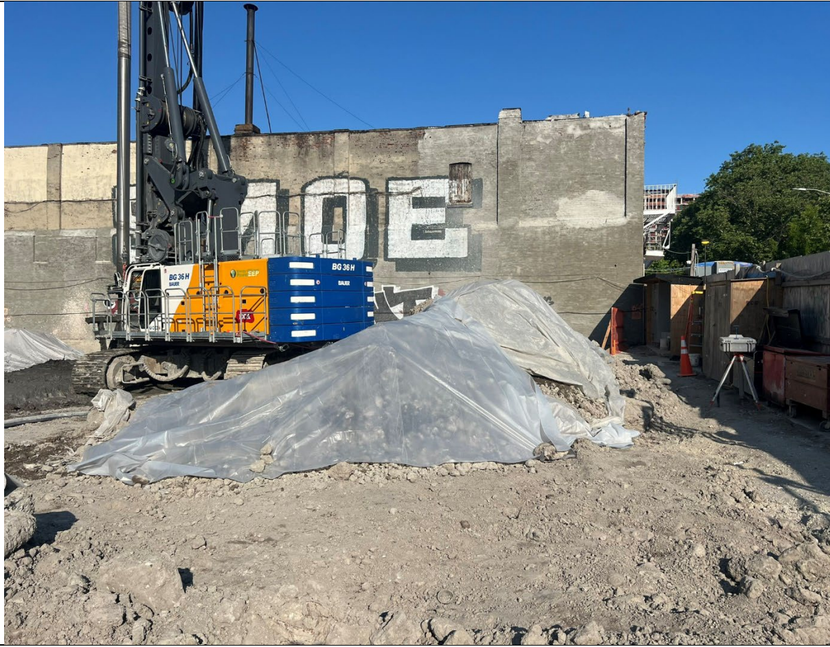
Photo 3- Representative photo of stockpile covered at the end of the day
