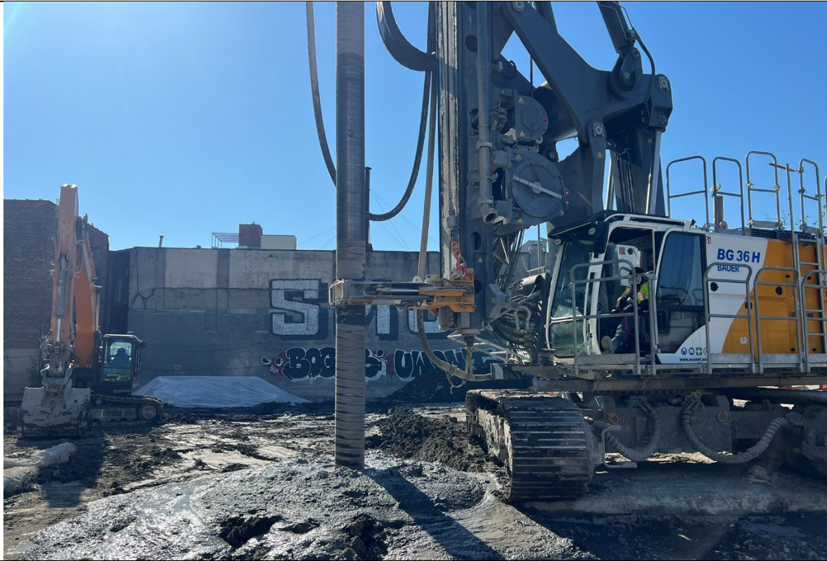
Photo 1- Representative photo of drilling an ISS column.
