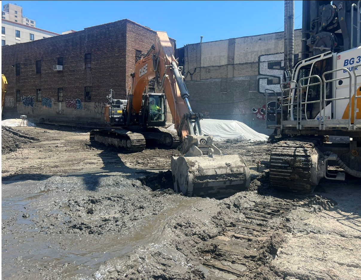
Photo 2- Representative photo of removing a shallow obstruction.
