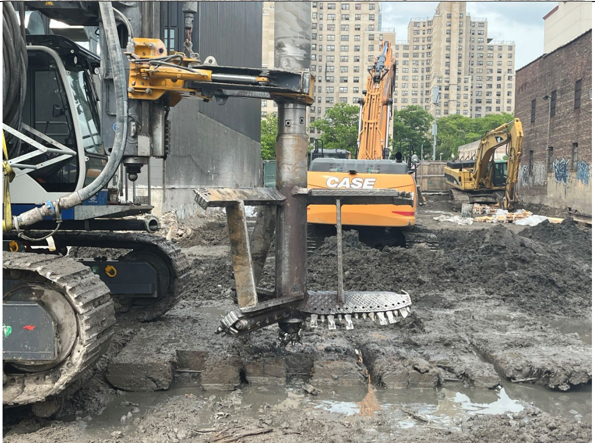
Photo 2- Representative photo of auger after decon.
