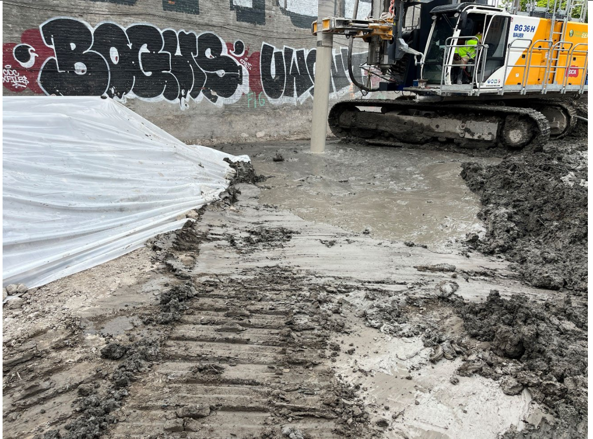
Photo 1- Representative photo of drilling ISS column.
