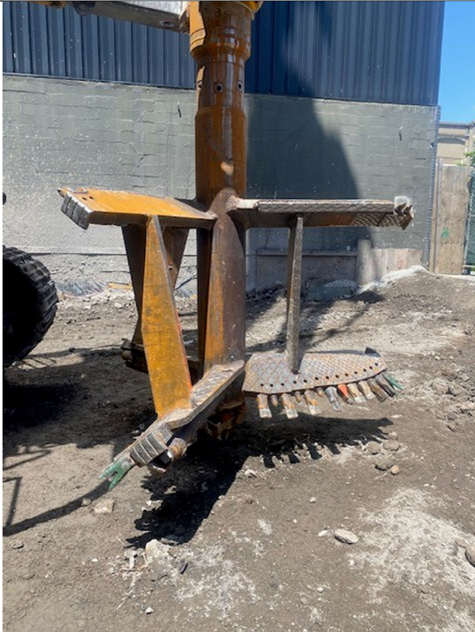
Photo 1- Representative photo of augur during maintenance.
