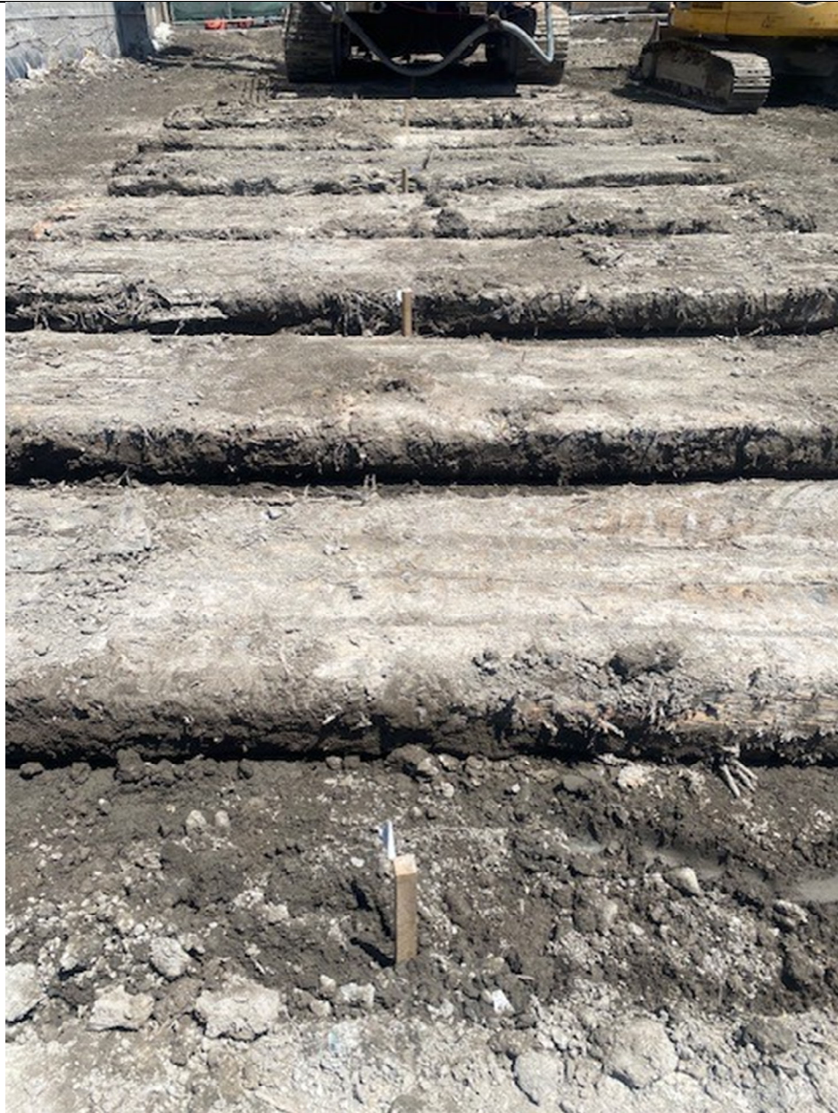
Photo 2- Representative photo of timber mats after relocation .
