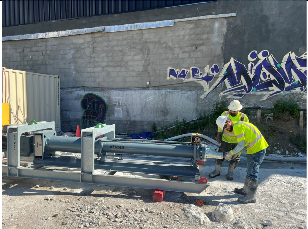
Photo 5- Representative photo of new pump being connected.
