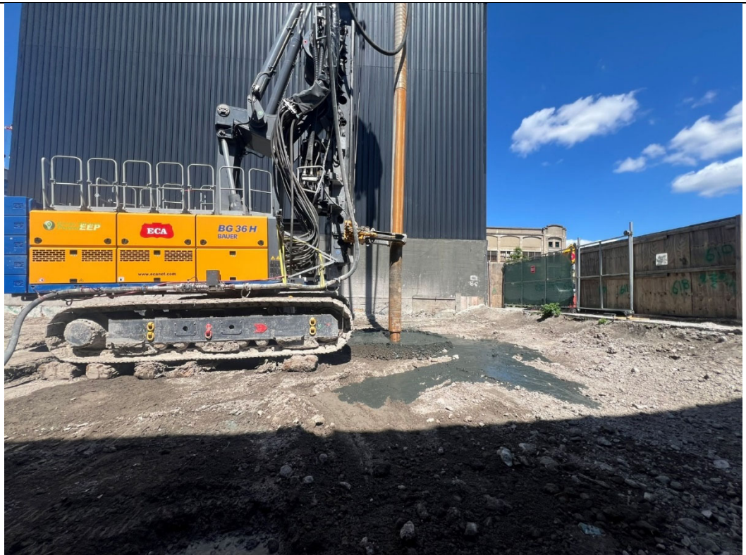
Photo 4- Representative photo of ISS column being installed.
