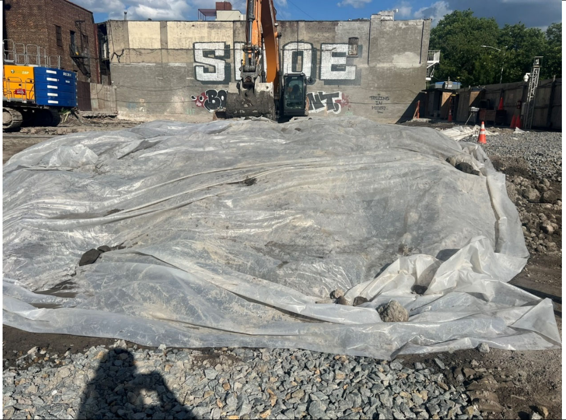
Photo 3- Representative photo of stockpile covered at the end of the day.
