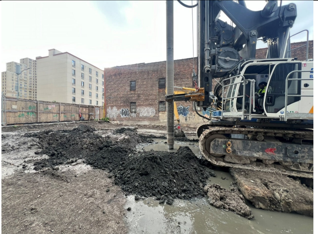
Photo 4- Representative photo of ISS column being installed.
