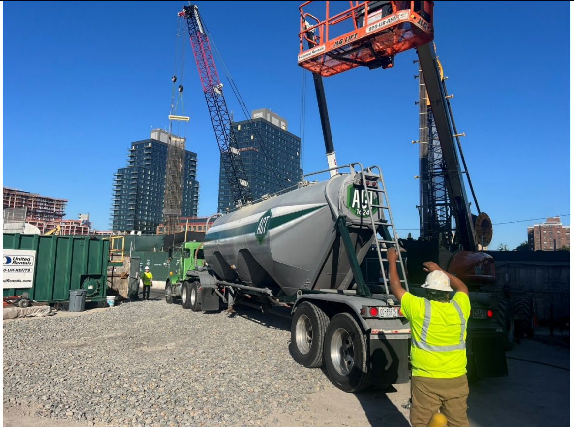
Photo 1- Representative photo of a slag delivery.
