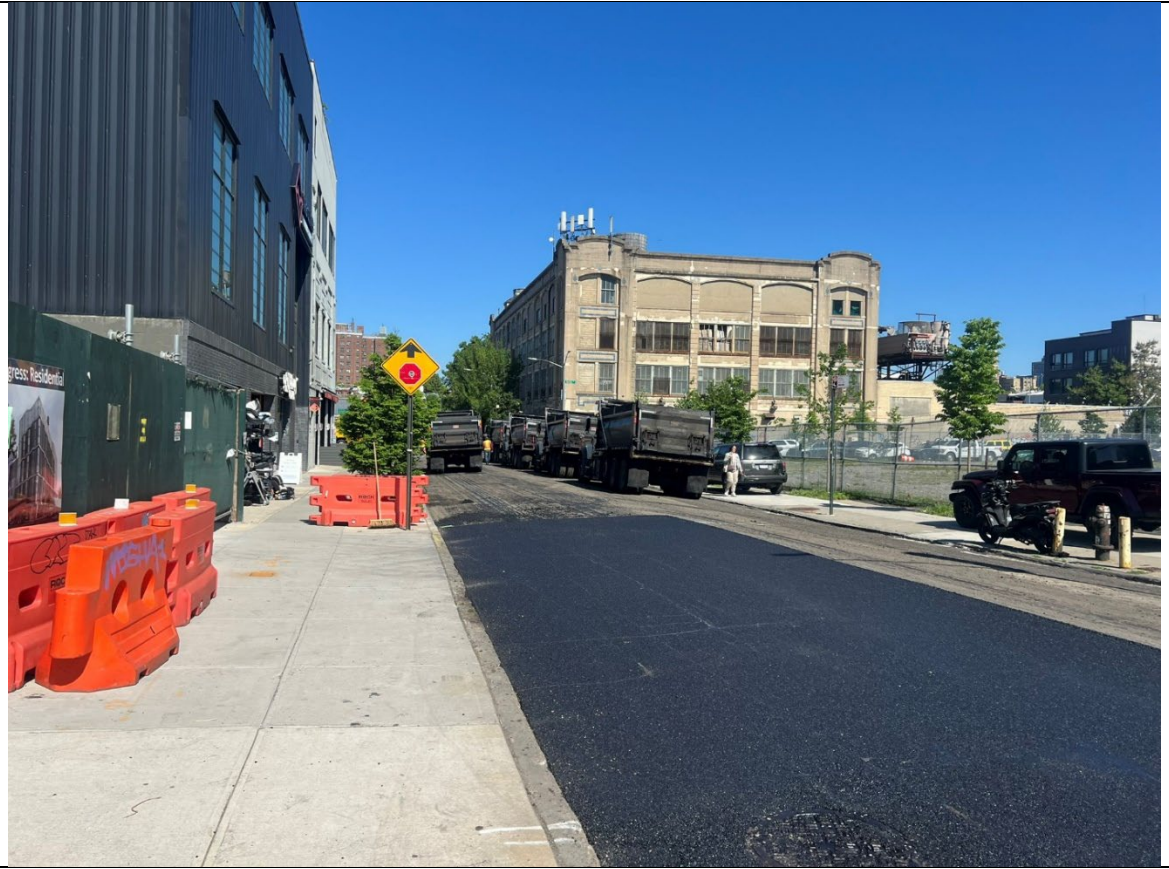
Photo 5- Representative photo of Butler Street being repaved.
