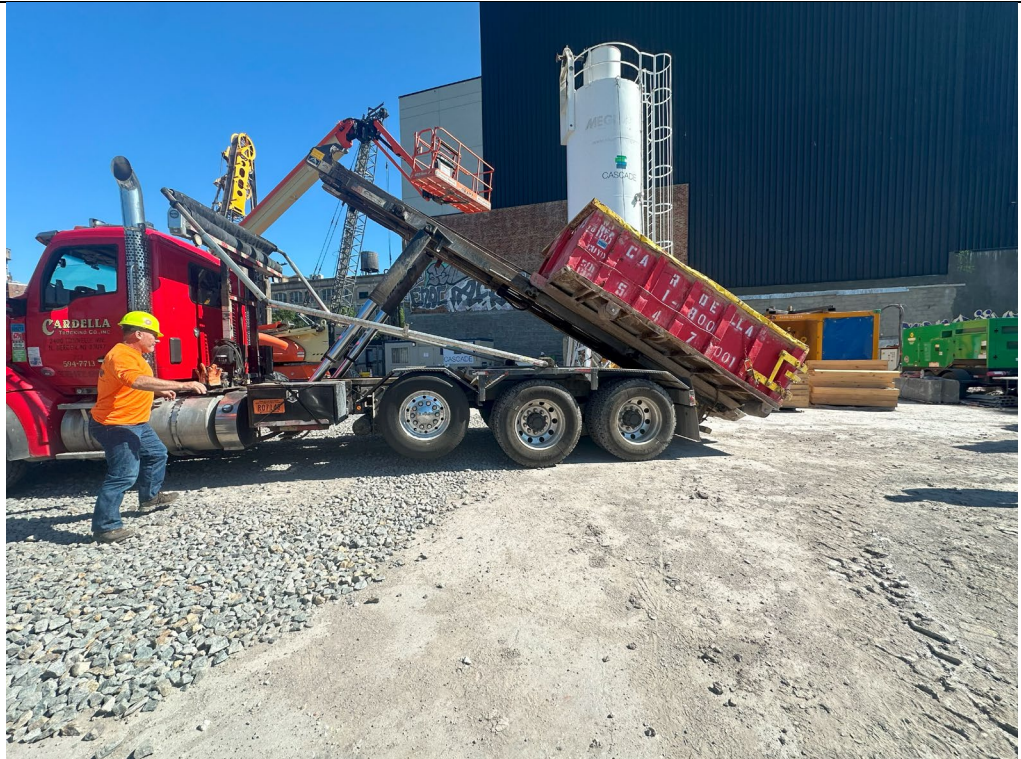
Photo 3- Representative photo of Cardella dropping off empty dumpster.
