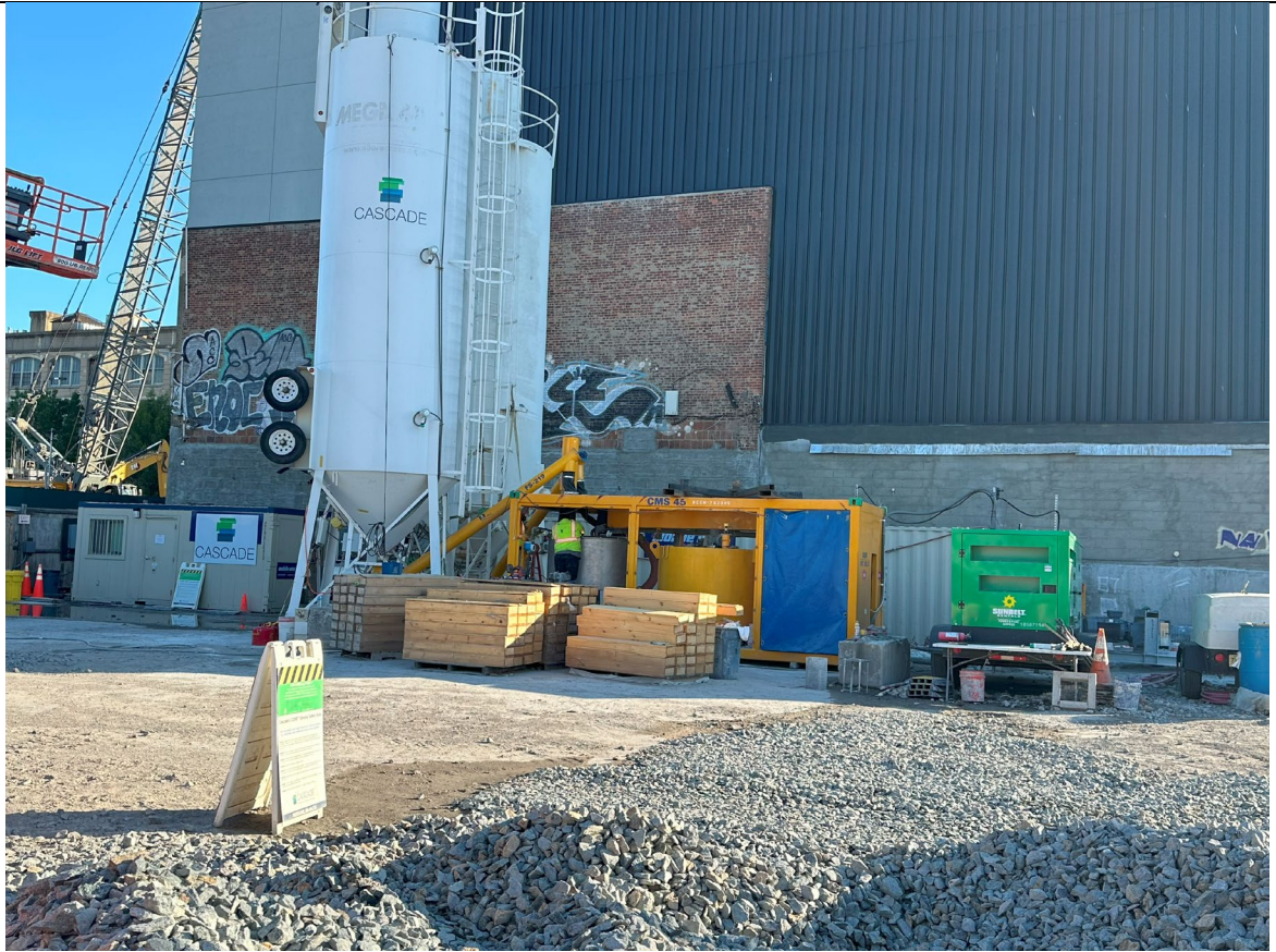
Photo 1- Representative photo of cascade crew cleaning batch plant.
