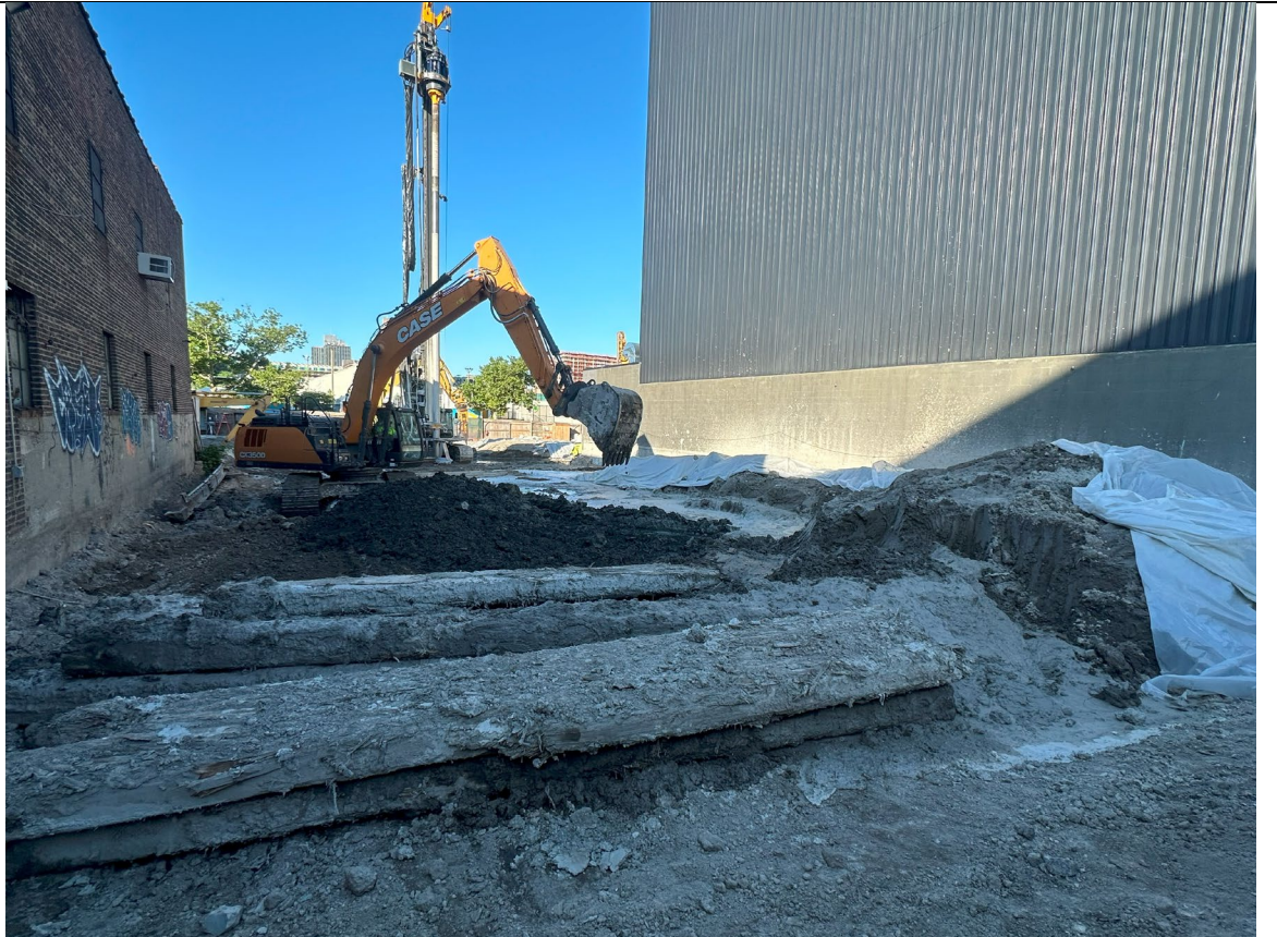
Photo 2- Representative photo of swell material being moved to stockpile.
