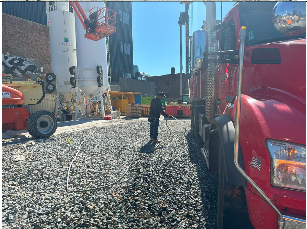
Photo 4- Representative photo of truck tires being washed over track pad.
