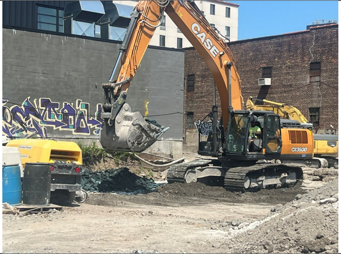
Photo 3- Representative photo of site maintenance.
