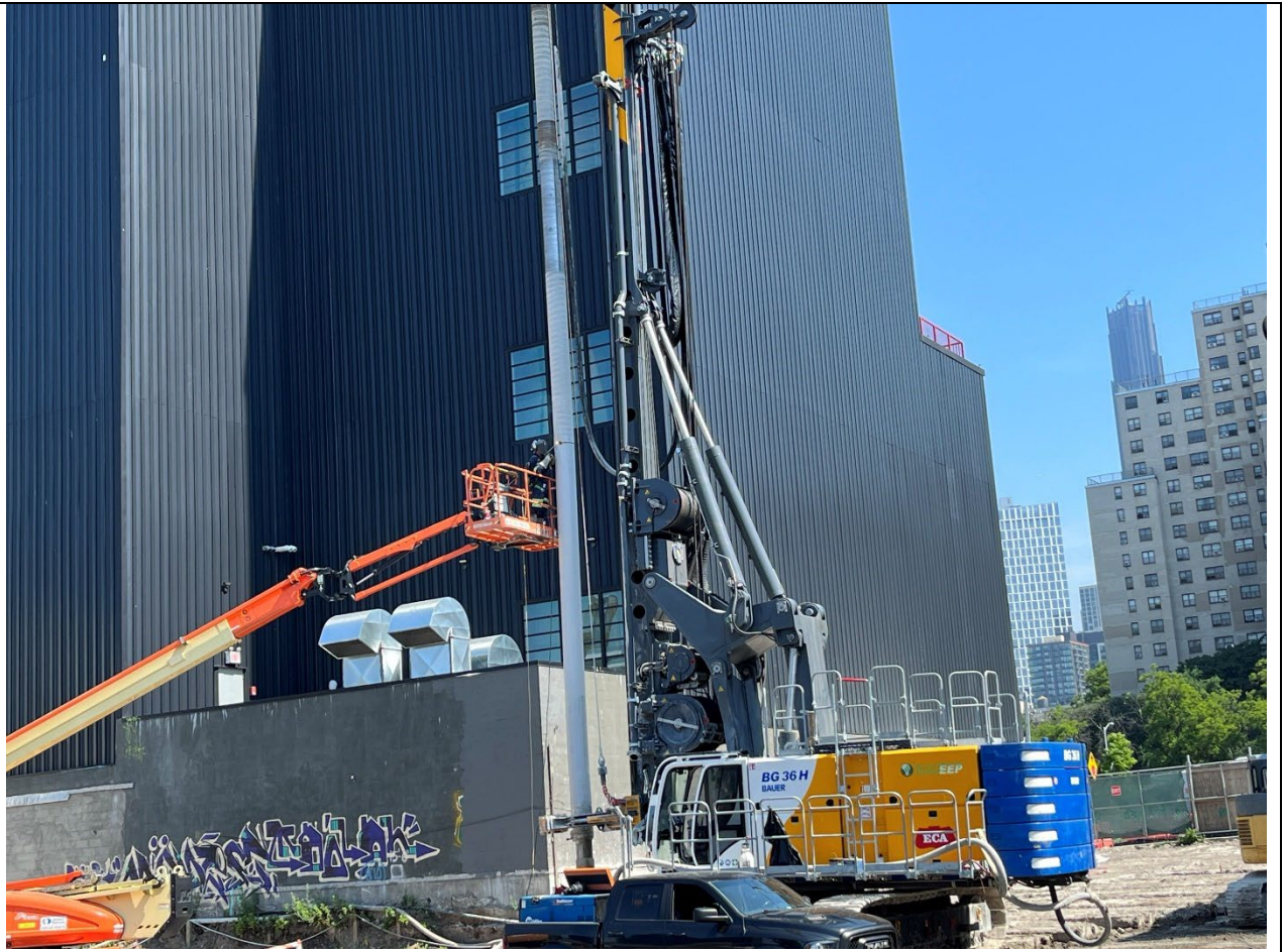
Photo 5- Additional photo of ECA performing Kelly Bar repairs.
