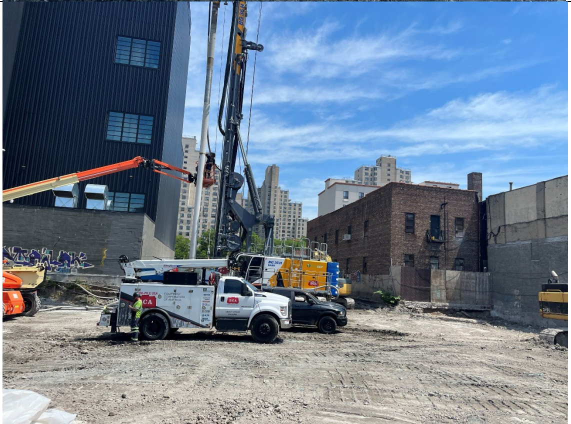
Photo 4- Representative photo of ECA performing Kelly Bar repairs.
