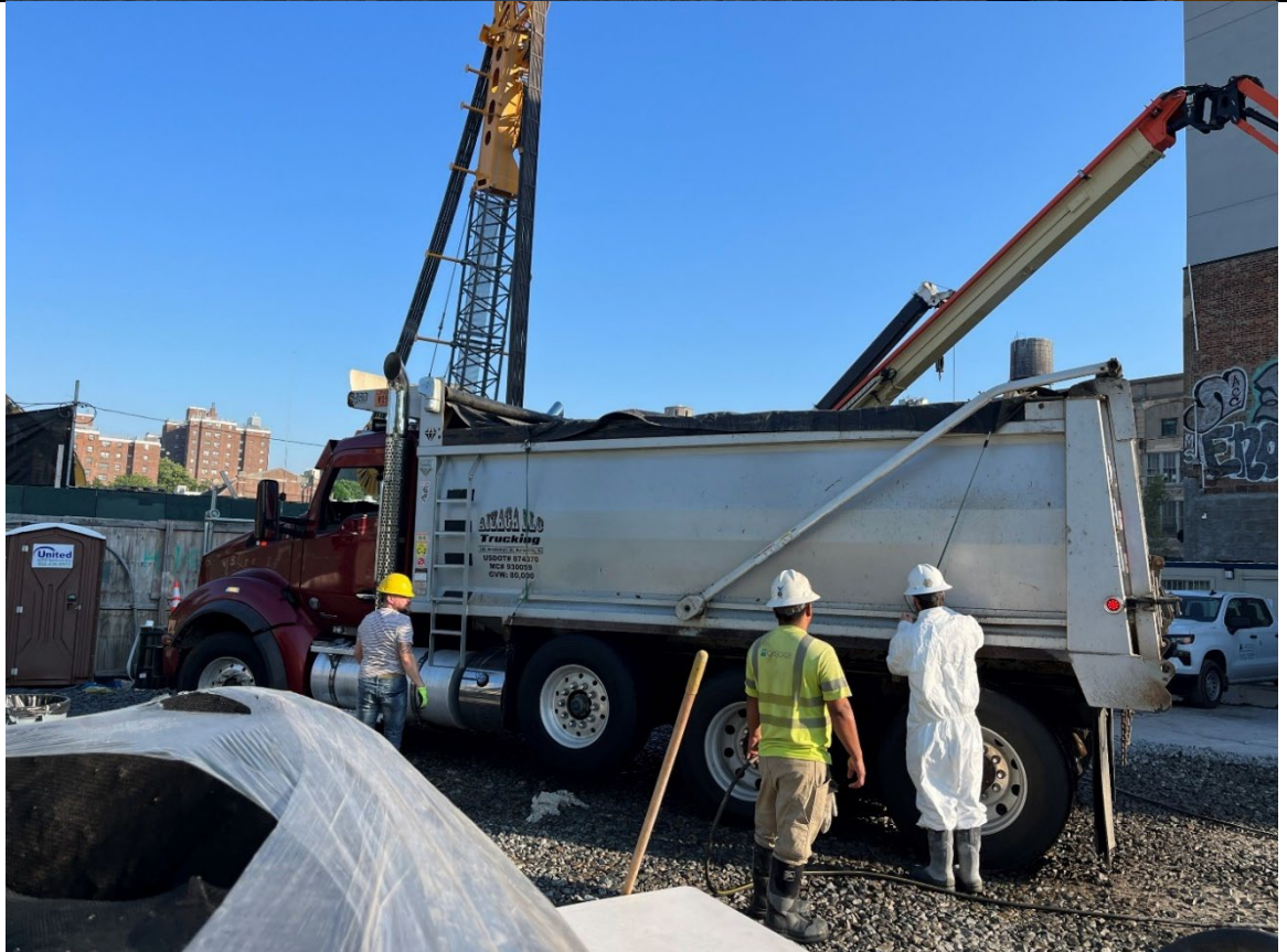
Photo 2- Representative photo of tarp strapped down on truck prior to truck exiting the Site.
