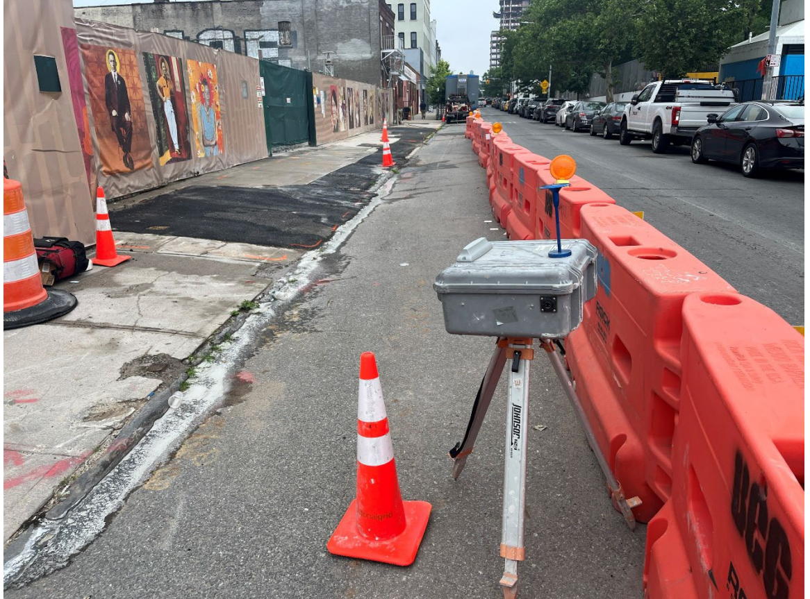
Photo 2- Representative photo of National Grid Work along Douglass Street.
