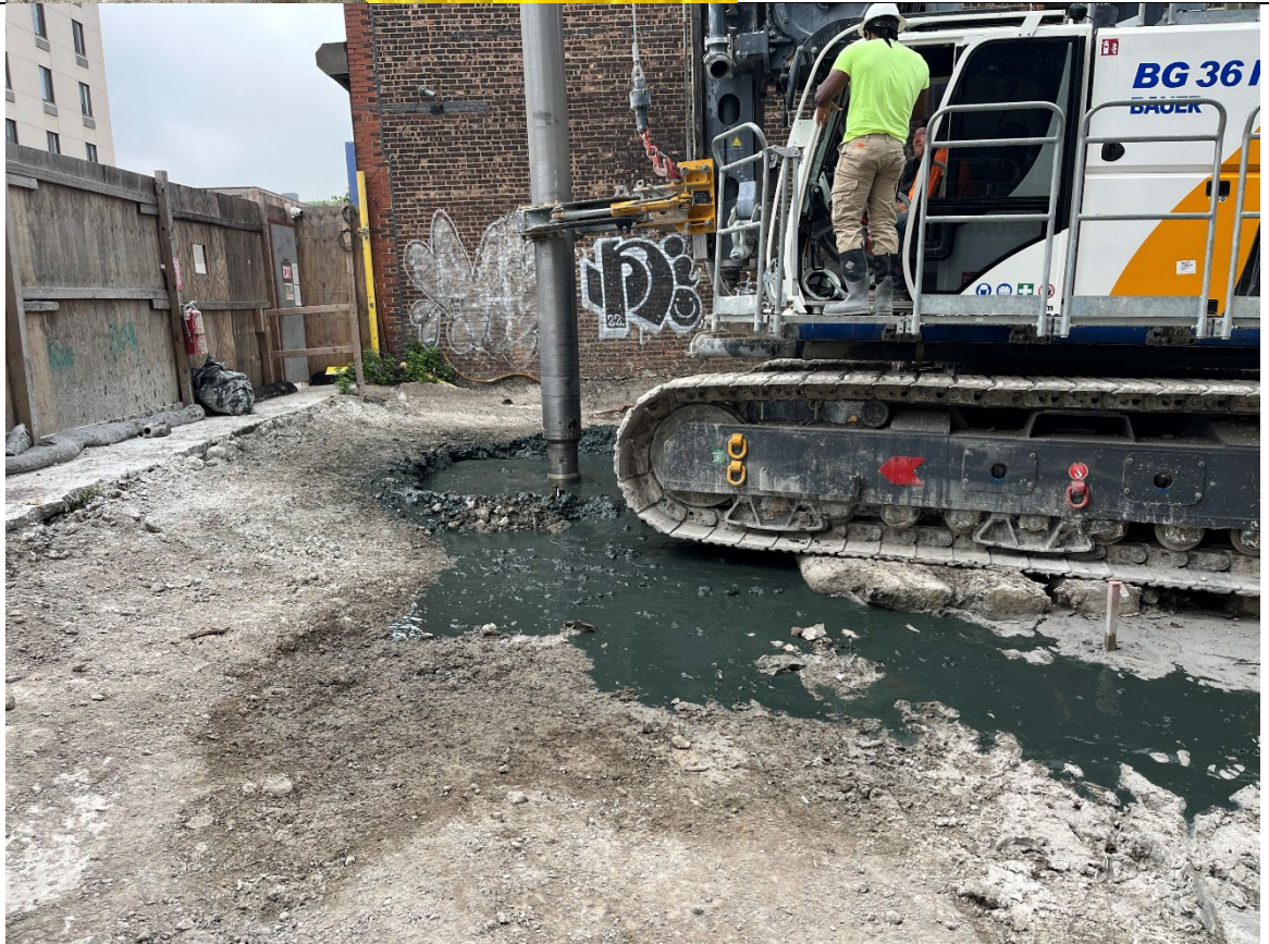
Photo 4- Representative photo of ISS column installation.
