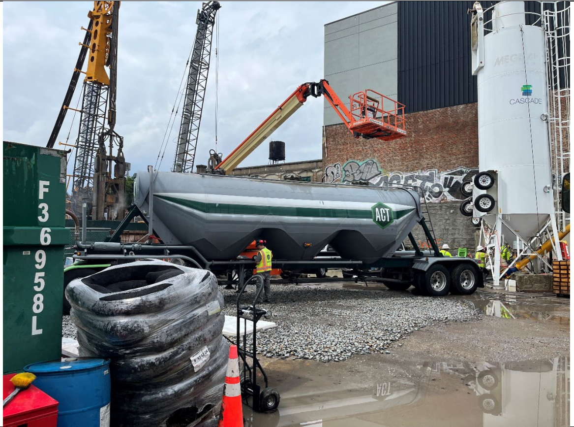
Photo 1- Representative photo of a slag delivery.
