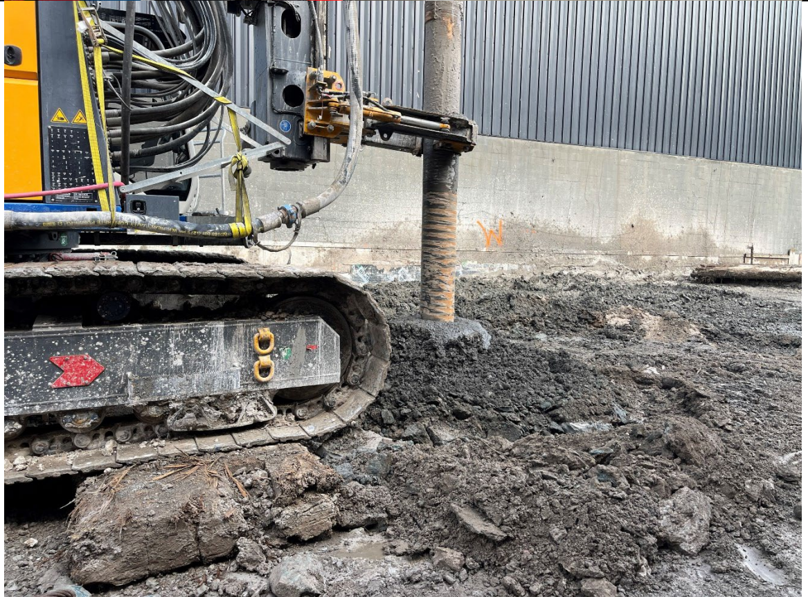
Photo 2- Representative photo of ISS column installation.
