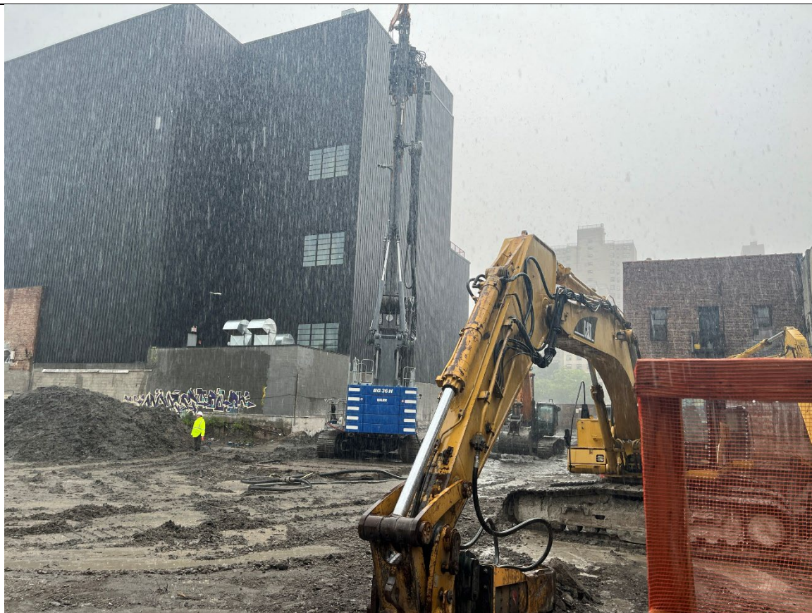
Photo 3- Representative photo of Site work facing north.
