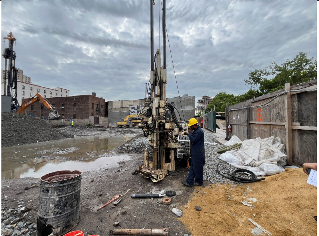
Photo 2- Representative photo of GES coring.
