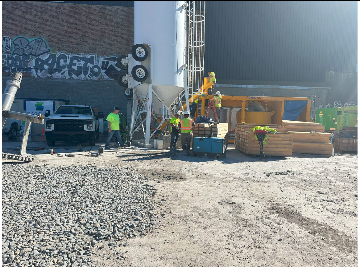
Photo 1- Representative photo of batch plant being clean and serviced.
