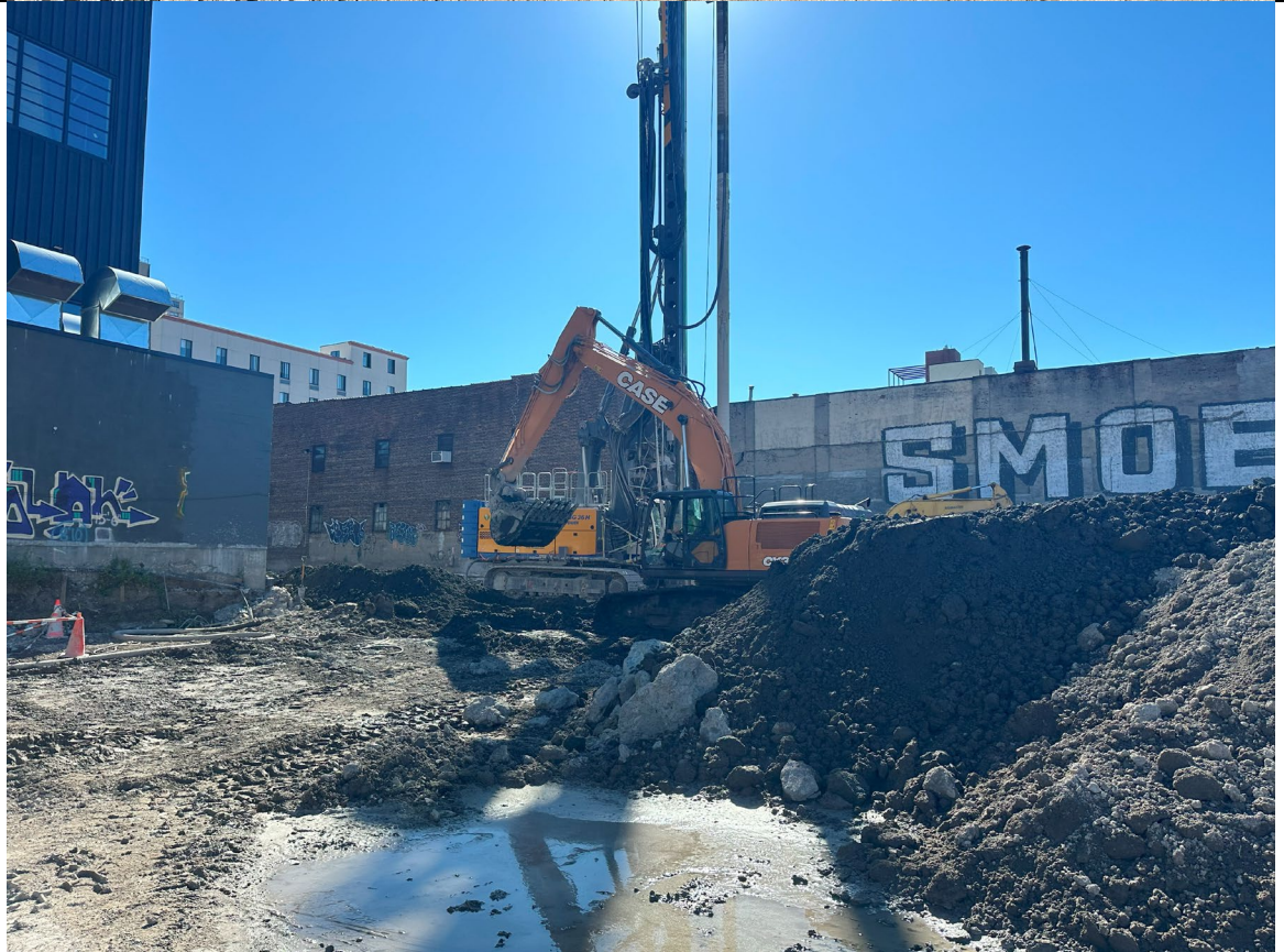
Photo 2- Representative photo of ISS swell being moved to stockpile.
