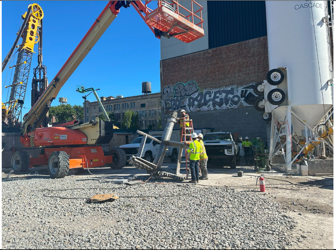
Photo 3- Representative photo of equipment maintenance.
